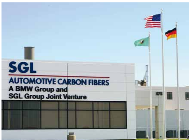
Groundbreaking in July 2010, completed only one year later: the plant in Moses Lake
