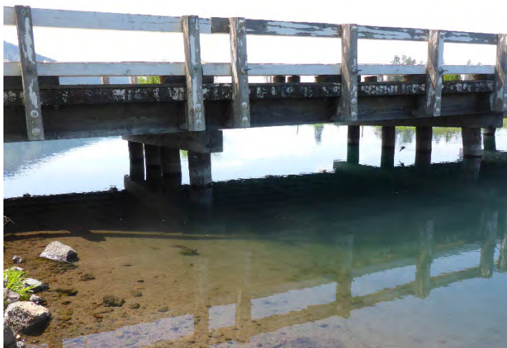
Photo 4.4-5. Existing bridge railing.
