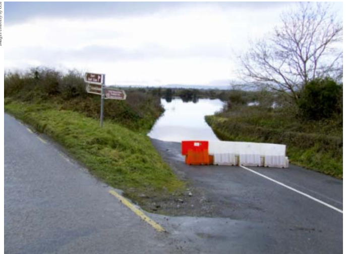
Road closure due to groundwater flooding, Gort Lowlands, Co. Galway.
