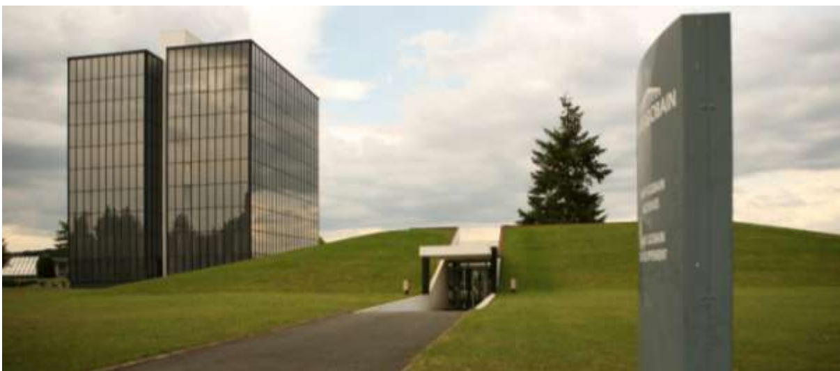
Image 1 – Exterior of the Saint-Gobain Archives (Photograph: Alain Dovifat)
