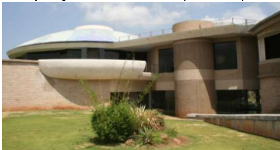
Image 1 – Building under construction that will house the Godrej Archives
