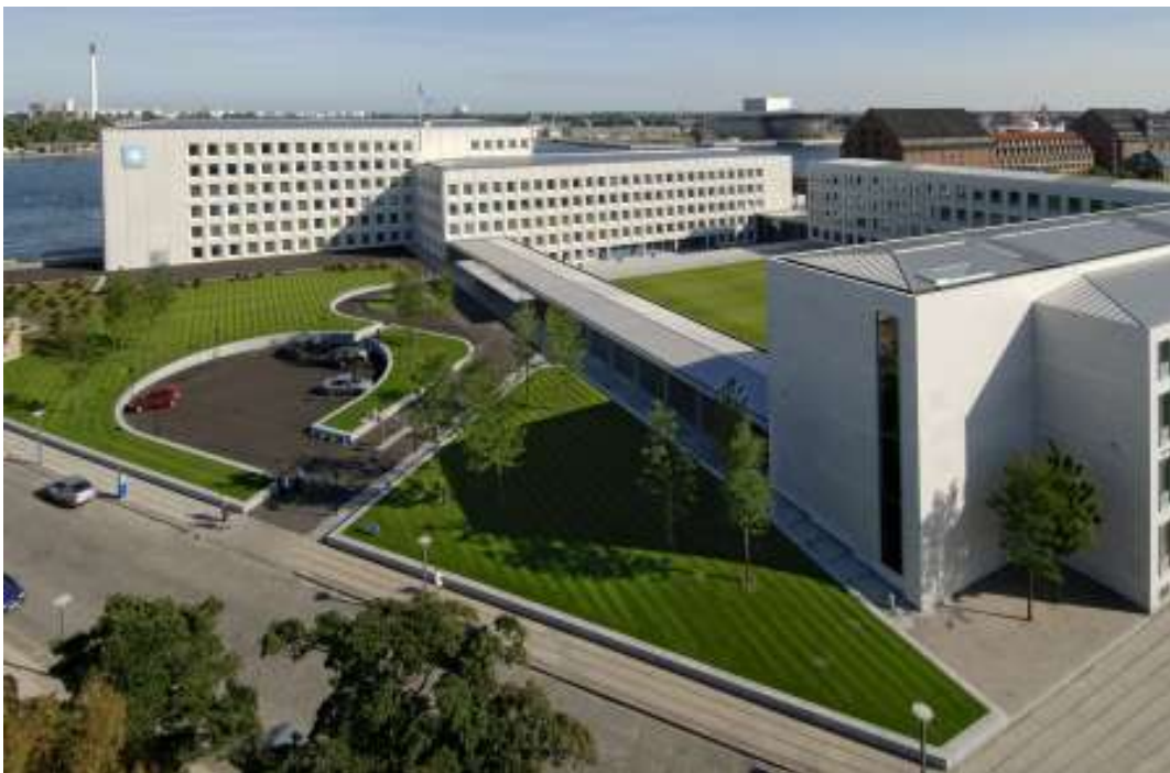
Image 2 – A.P. Møller – Mærsk Headquarters, Copenhagen, Denmark
