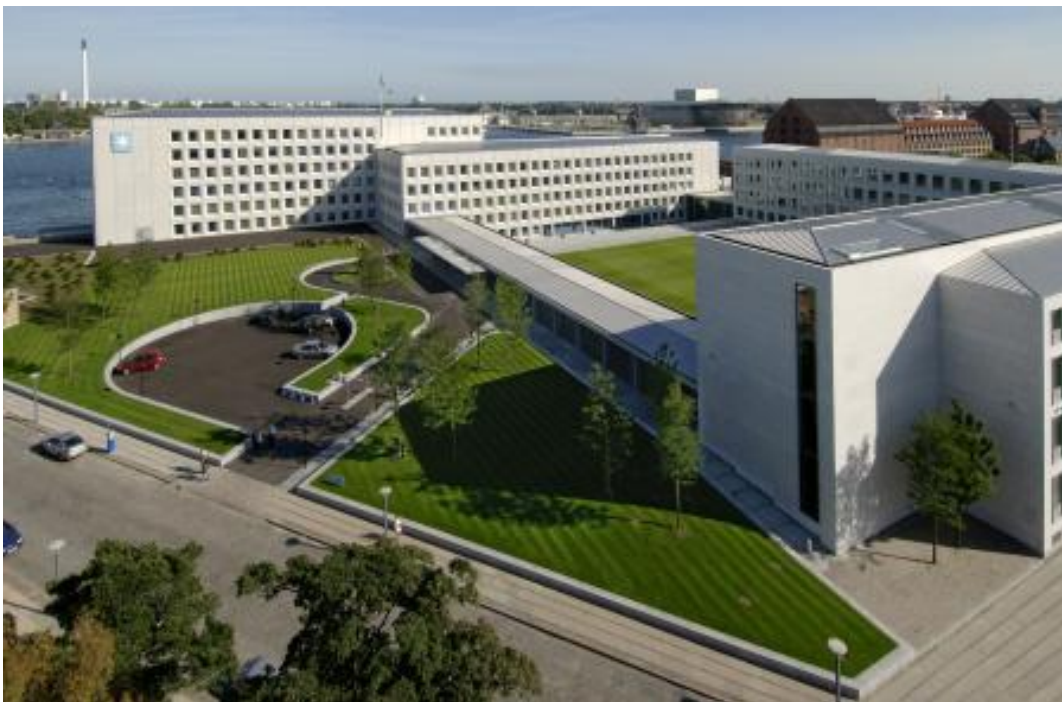
Image 2 – A.P. Møller – Mærsk Headquarters, Copenhagen, Denmark
