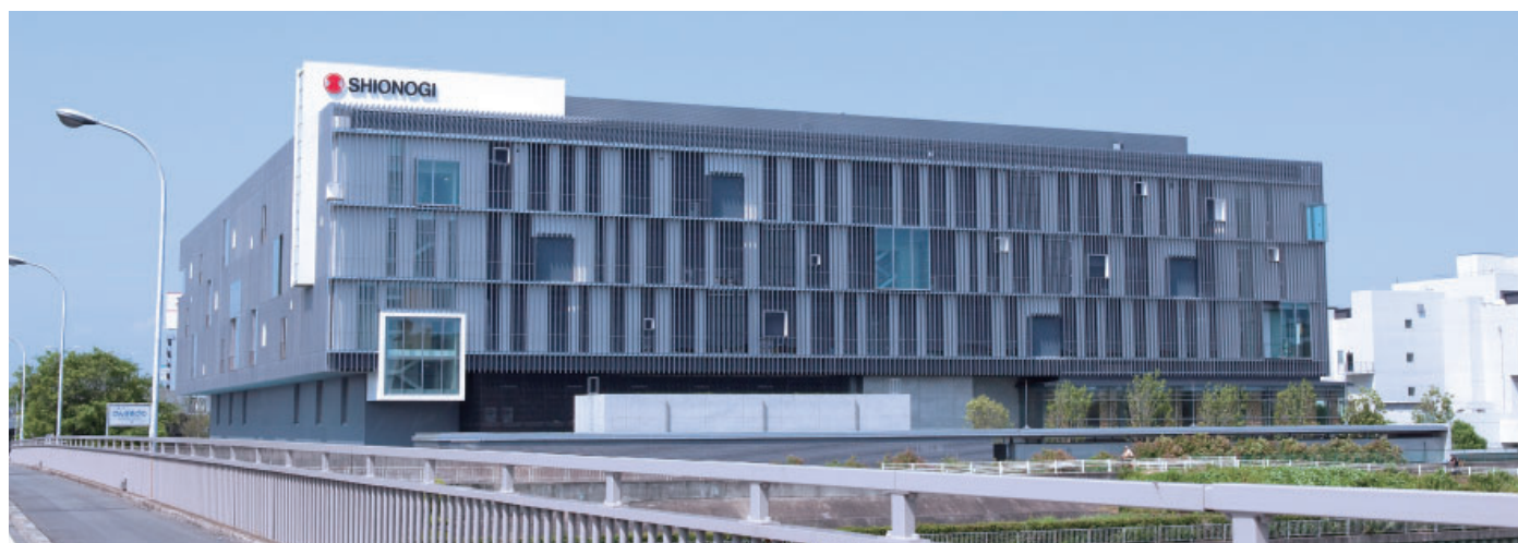
The new pharmaceutical research building was completed in July 2011
