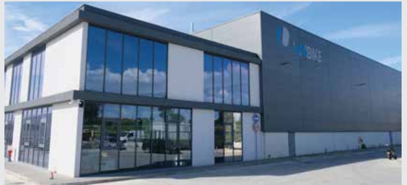
Construction of the new headquarters of Unibike was finished in the spring of 2021.
