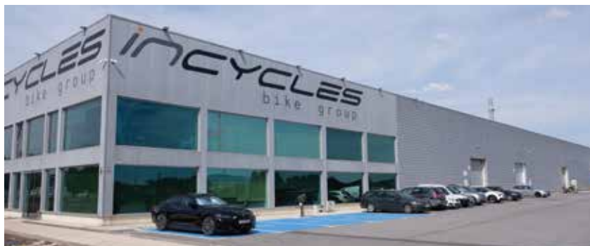
Formerly a factory for motorbikes, the headquarters of In Cycles have been purposed for the assembly of e-bikes
