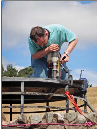
Below: Ian drilling mounting holes for the MCRO Larkin frame.
