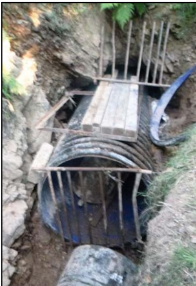
Above: The old gate used as a grill on the new pipe in the entrance to Yew Tree level, fitted on the 19th July.
