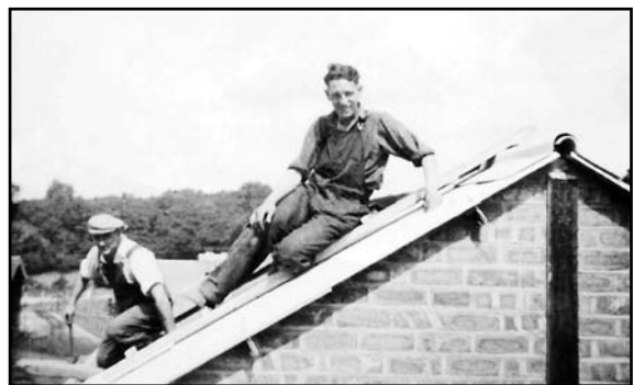
George Poyner (right) and fellow carpenter, Harry Deakin (left) roofing the dirt disposal shed at Alveley. ( George Poyner Collection )
