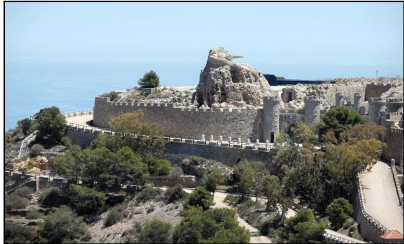
Above: Distant view of the gun battery on Cabo Tinoso.
