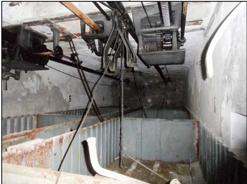
Above: Overhead shell handling equipment to fetch shells which were stored in the tanks.
