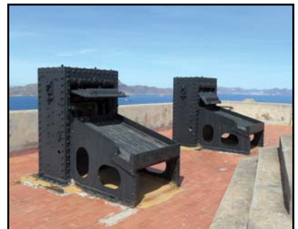
Below: Top end of the 6" shell feeders just behind the guns.
