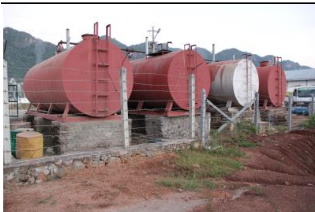
Figure 9.8 Fuel Storage Area at the Cement Plant
