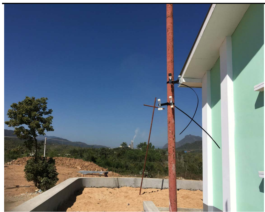
Figure 6.2 Air Quality Monitoring Station at AQ1: Worker Accommodation Quarters
