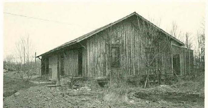
Railroad freight-house located on the same development site with the gasholder house. Photo courtesy of David Perrotta.
