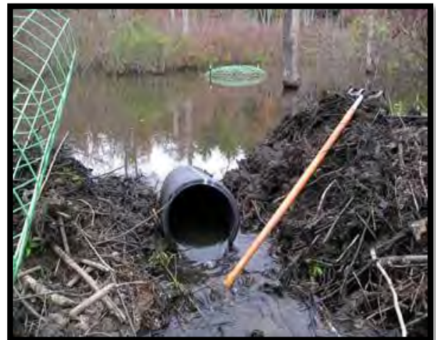
Figure 35: Flexible pond levelers with cylindrical wire cages on the upstream pipe end. Clockwise from upper left (a) and (b) are examples during the construction phase, while (c) is an example just after completion but before dam repair. (b) is a downstream view of a pond leveler after beaver have repaired the dam. Photographs from Boyle (2006).
