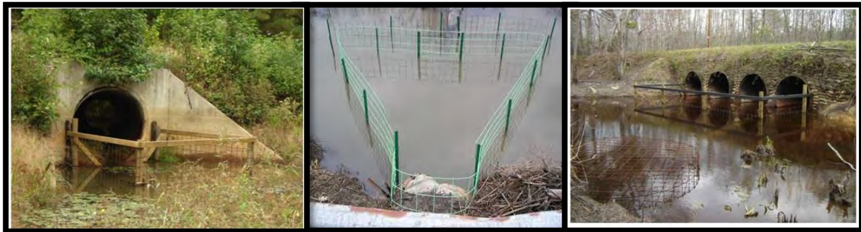
Figure 38: Examples of culvert-protective fences. From left to right: (a) and (b) are stand-alone culvert-protective fences, while (c) is a stand-alone fence combined with a flexible pond leveler pipe (underwater and not visible) and a cylindrical wire mesh cage, which provides extra protection against obstruction. Figures from Boyle (2006).
