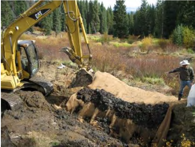
Figure 62: Breached dams were “plugged” with soil lifts wrapped in coir fabric and sod interwoven with live willow stems
