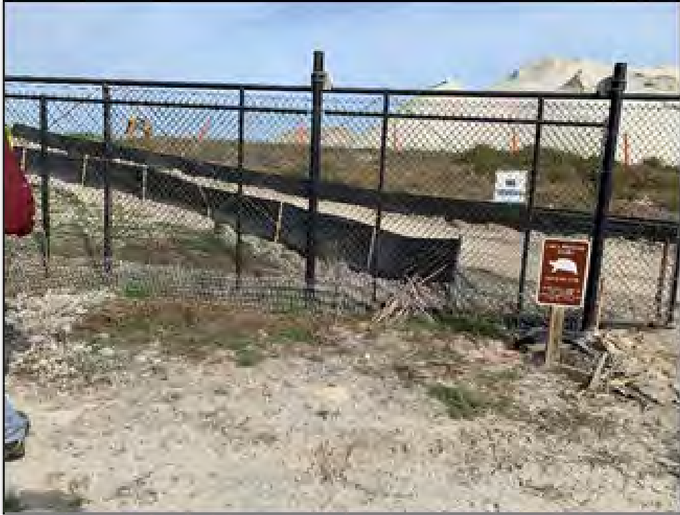
Figure 3. Preparation & Installation of Exclusionary Devices (January 7, 2021)
