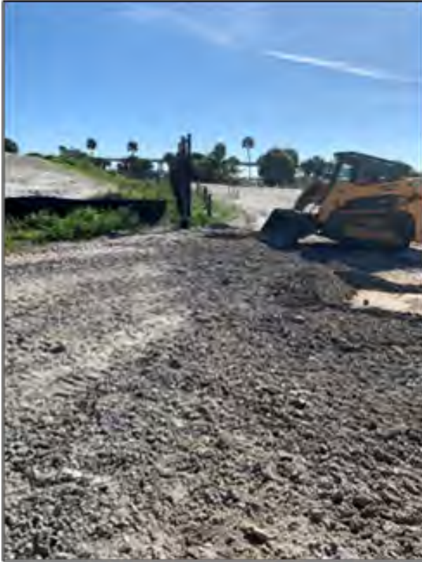
Figure 6. Re-grading at Main DMMA Entrance Gate
