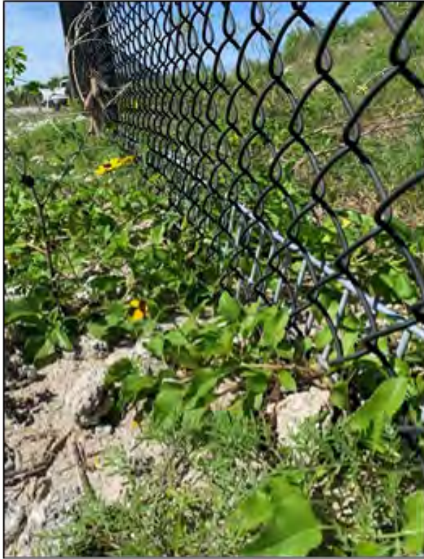
Figure 5. Installation Complete, January 8, 2021
