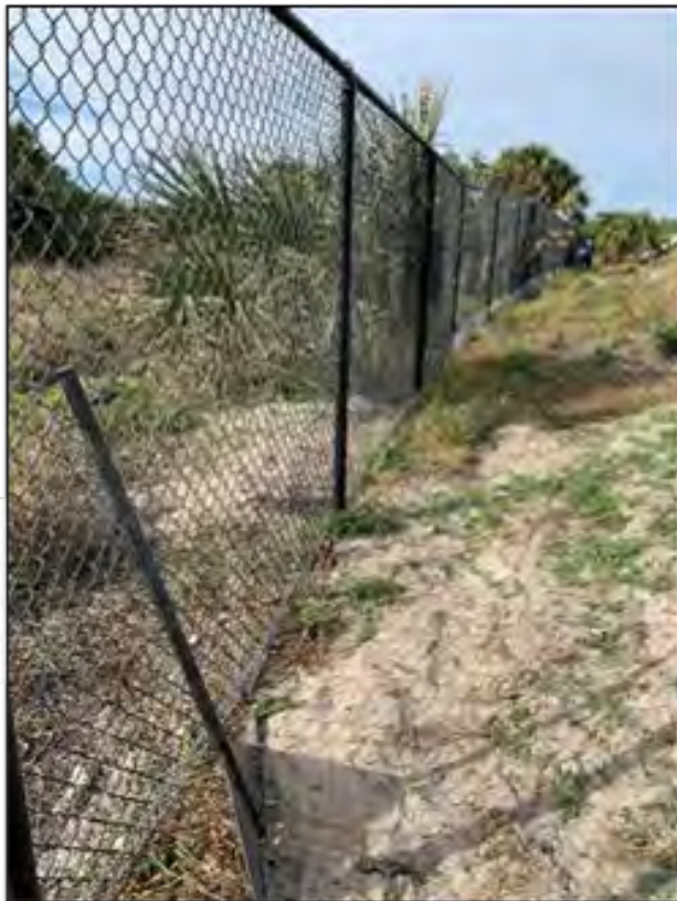
Figure 4. Dig Defence® to remain Approximately three (3) inches above ground elevation and woven into the existing fence structure
