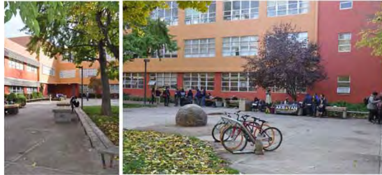
View south into courtyard of the Art Building
