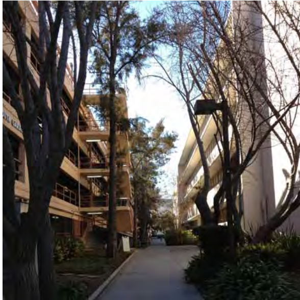
View looking west between the S. Parking Garage and Sweeney Hall
