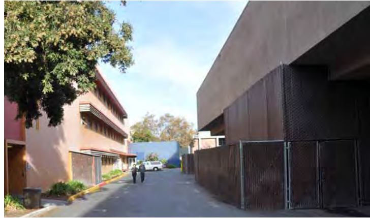
View looking east past Art Building and Event Center towards 9th Street Mall
