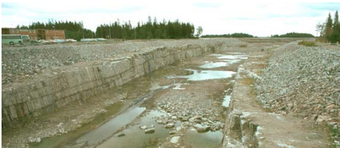
Figure 7-3. The channel between the nuclear power reactors and the Baltic Sea exposing extensive undulating sheet joints. Photograph by G Hansson. Reproduced from Carlsson and Christiansson (2007).
