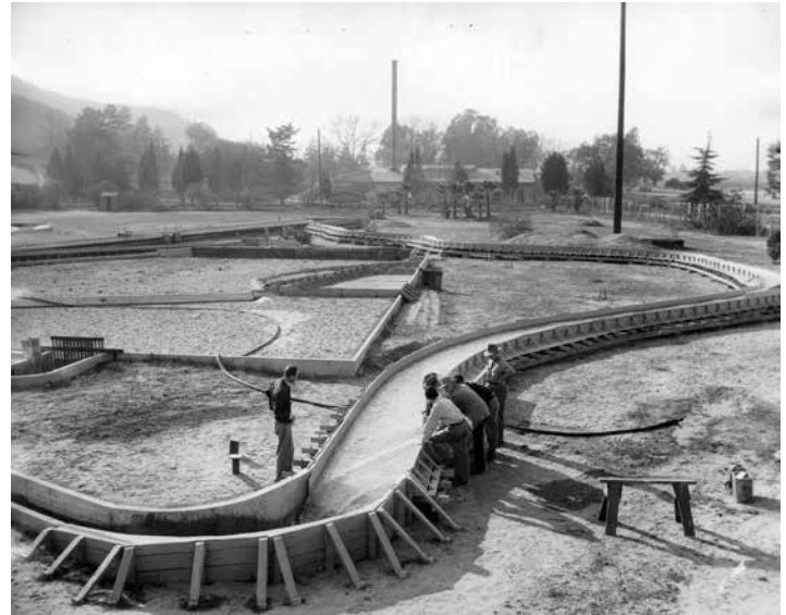
This 1948 image shows the US Army Corps of Engineers' open-air hydraulics laboratory in Griffith Park. The structures shown were built to model the Los Angeles River and proposed flood control facilities. Photo: Herald-Examiner Collection/Los Angeles Public Library.
