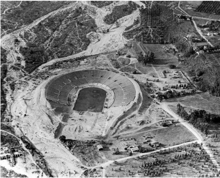
Rose Bowl stadium, shown above under construction in 1922 was built in the Arroyo Seco canyon of Pasadena. At the time of construction, the Arroyo Seco was still unchannelized and can be seen meandering through the canyon. Photo: Security Pacific National Bank Collection/Los Angeles Public Library.
