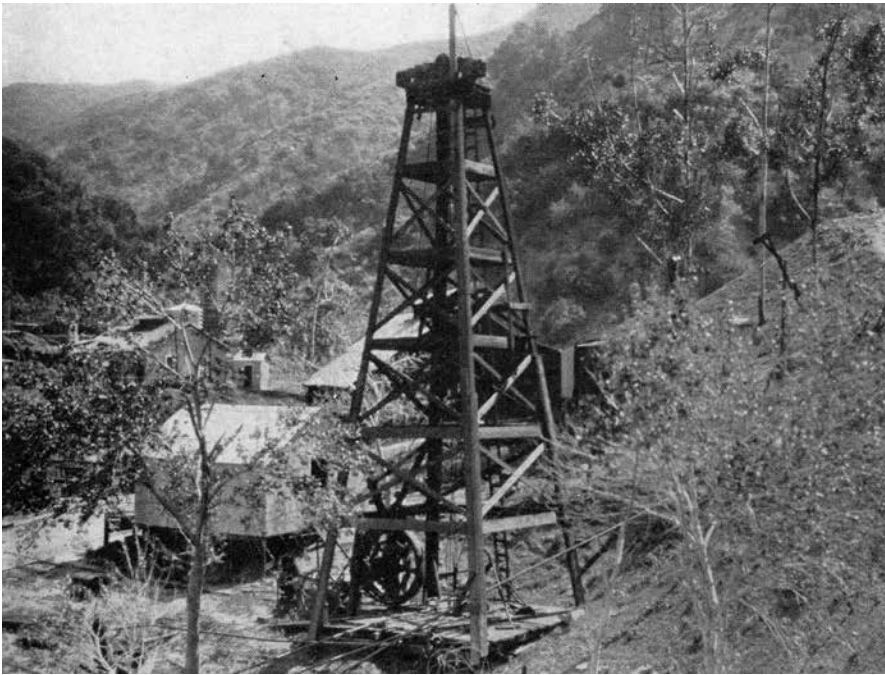
The newspaper caption to this 1931 photo of Well No. 4, Pico Canyon reads, "At the head of Pico Canyon, in the old Newhall oil field, stands this diminutive derrick known as the California Star Oil Works Company No. 4 well. It has faithfully produced for 54 years and is the oldest active well in California." Photo: Herald-Examiner Collection/Los Angeles Public Library.
