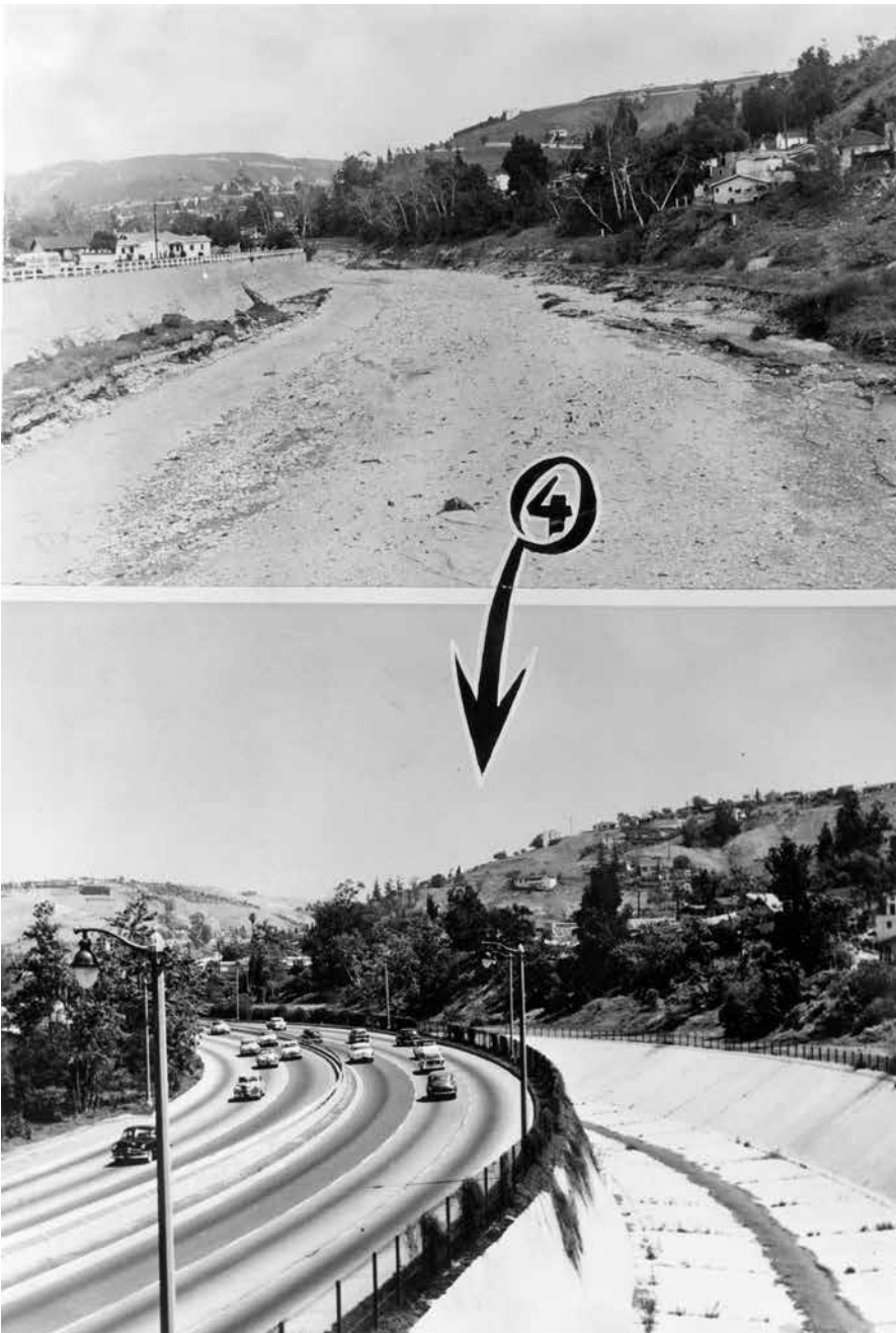
The first freeway in the west, the Arroyo Seco Parkway, was completed in 1940 in conjunction with channelization of the Arroyo Seco. This pair of photos illustrates the transformation of the Arroyo Seco from a natural waterway into the Arroyo Seco Parkway and adjacent flood control channel. Photo: Herald-Examiner Collection/Los Angeles Public Library.
