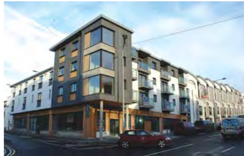
Apartments at Connaughton Road
