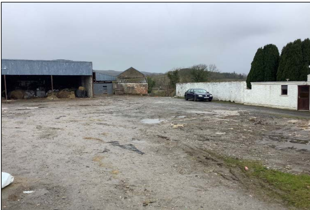
Plate 13-58 Route of proposed construction access road where it commences at the east, looking west.
