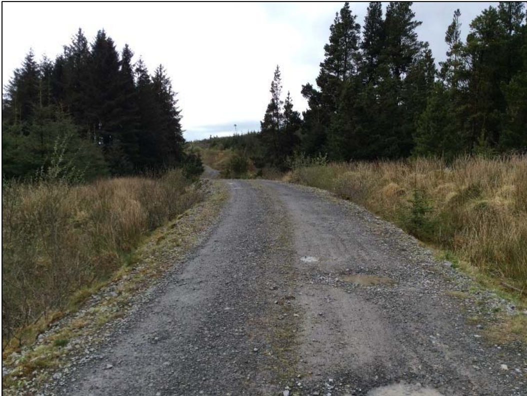
Plate 13-79 Entrance into core wind farm site looking north-west.
