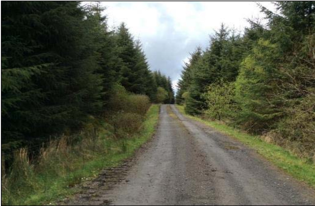
Plate 13-57 Route of proposed grid connection cable route looking west before it reaches the site of the proposed substation
