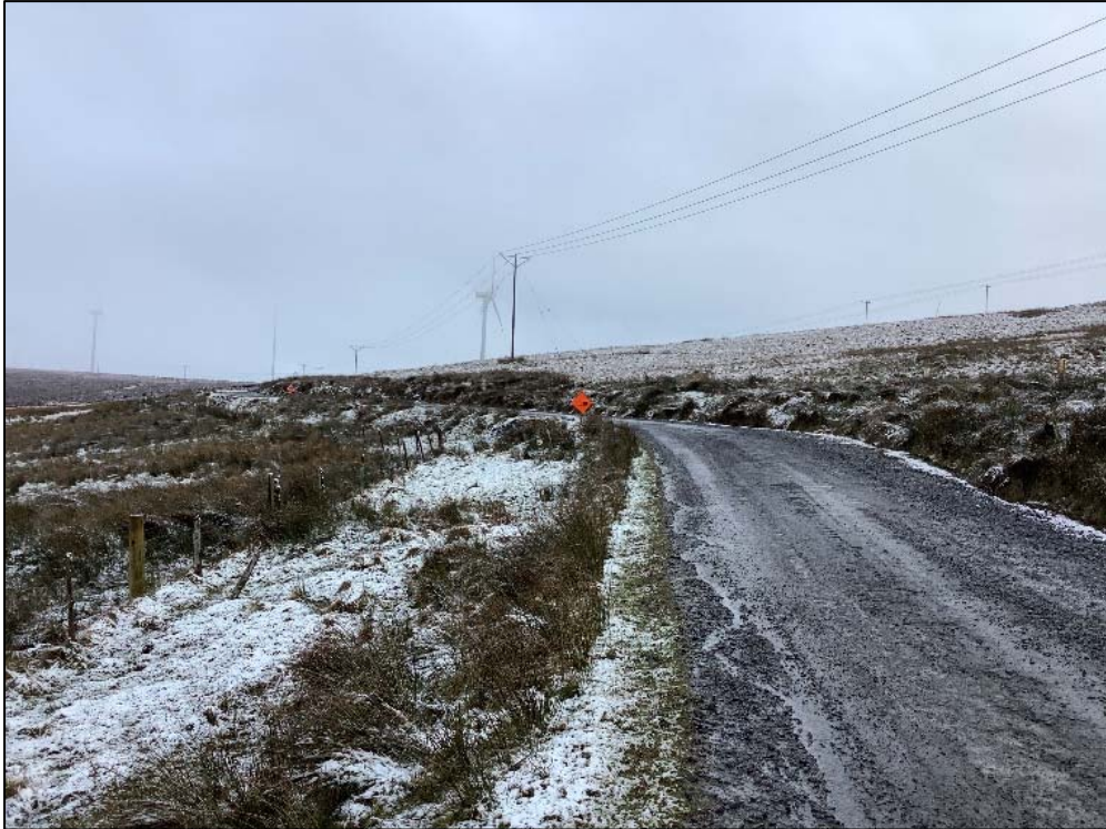
Plate 13-75 Proposed construction access road along existing road where upgrade works are proposed, looking south
