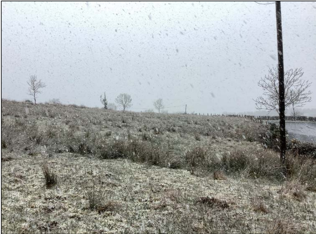
Plate 13-63 Continuation north of section of road widening at Derrycullinan Td.
