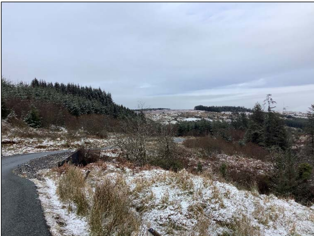
Plate 13-74 Continuation of proposed construction access road along public road (some road widening may be required here).
