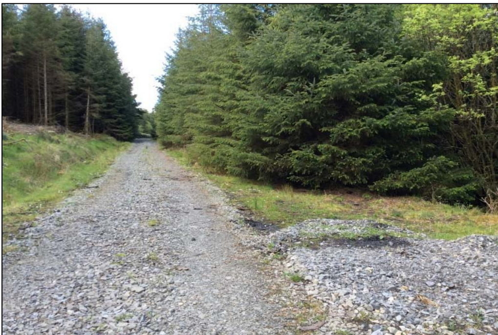
Plate 13-64 Section of proposed construction access road along existing road looking NW in Derrycullinan townland.
