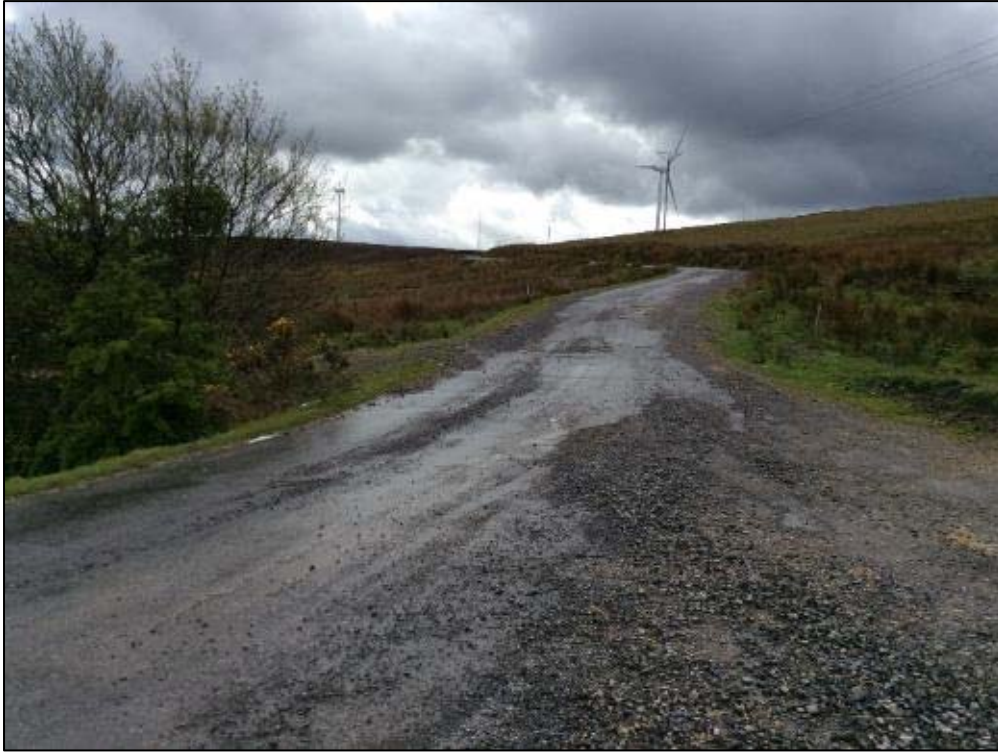
Plate 13-49 Existing road along grid connection cable route looking south
