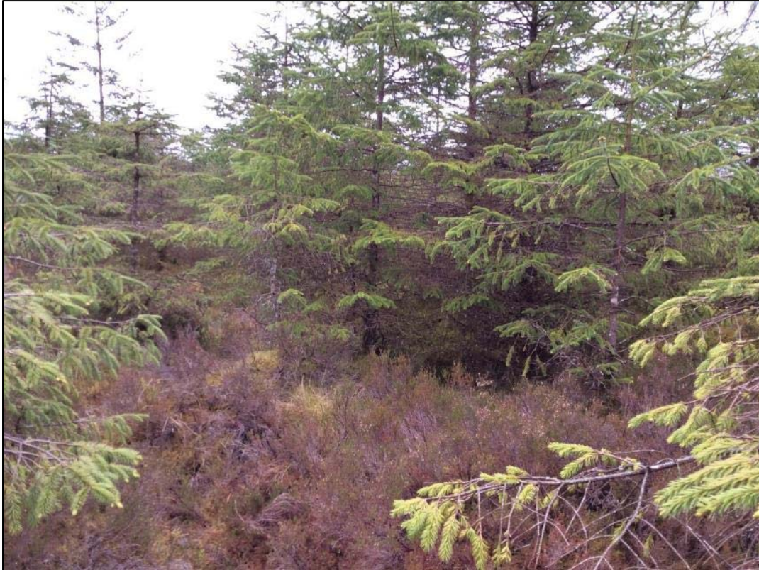
Plate 13-25 Continuation of new road through forestry looking south-east
