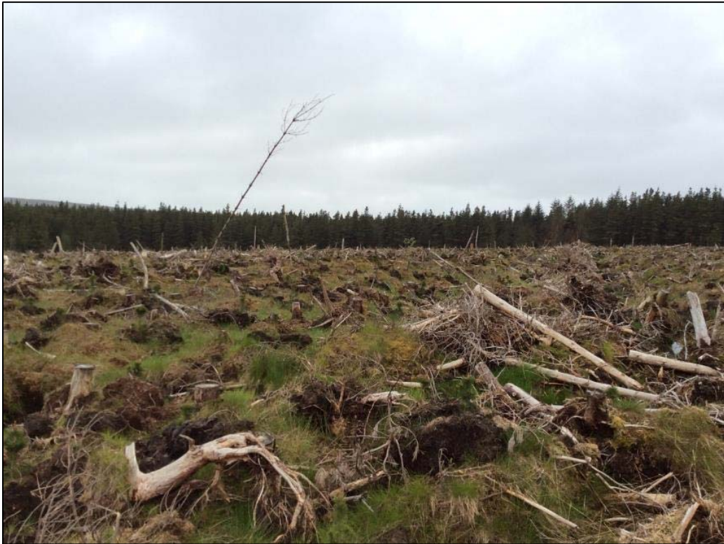
Plate 13-23 Hardstand of turbine 7 looking southwest.
