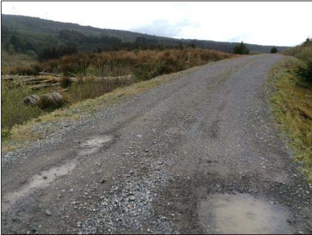
Plate 13-53 Continuation of proposed grid connection cable route looking north (within site boundary)
