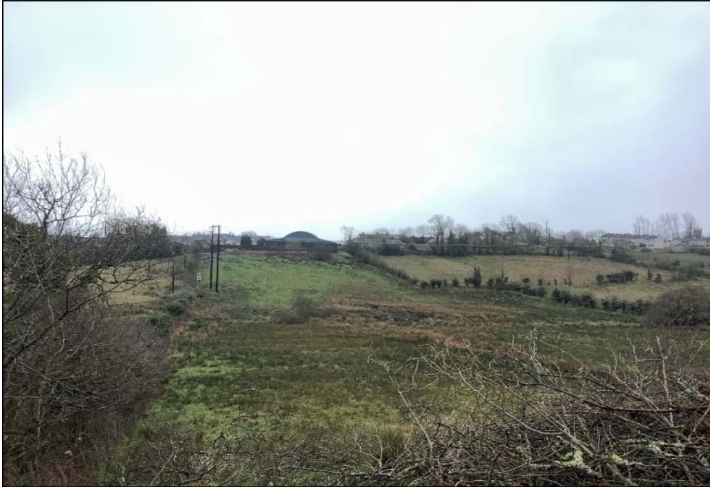
Plate 13-61 Construction access road from public road to west looking east towards agricultural sheds and Drumkeeran.
