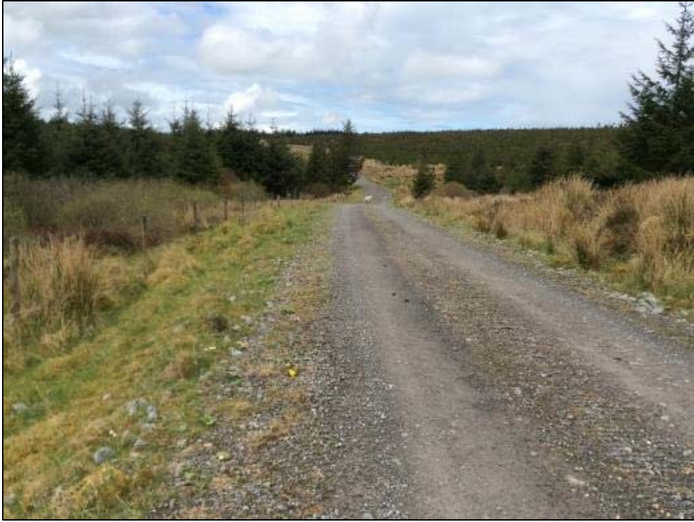
Plate 13-55 Continuation north of proposed grid connection cable route looking north (within site boundary)
