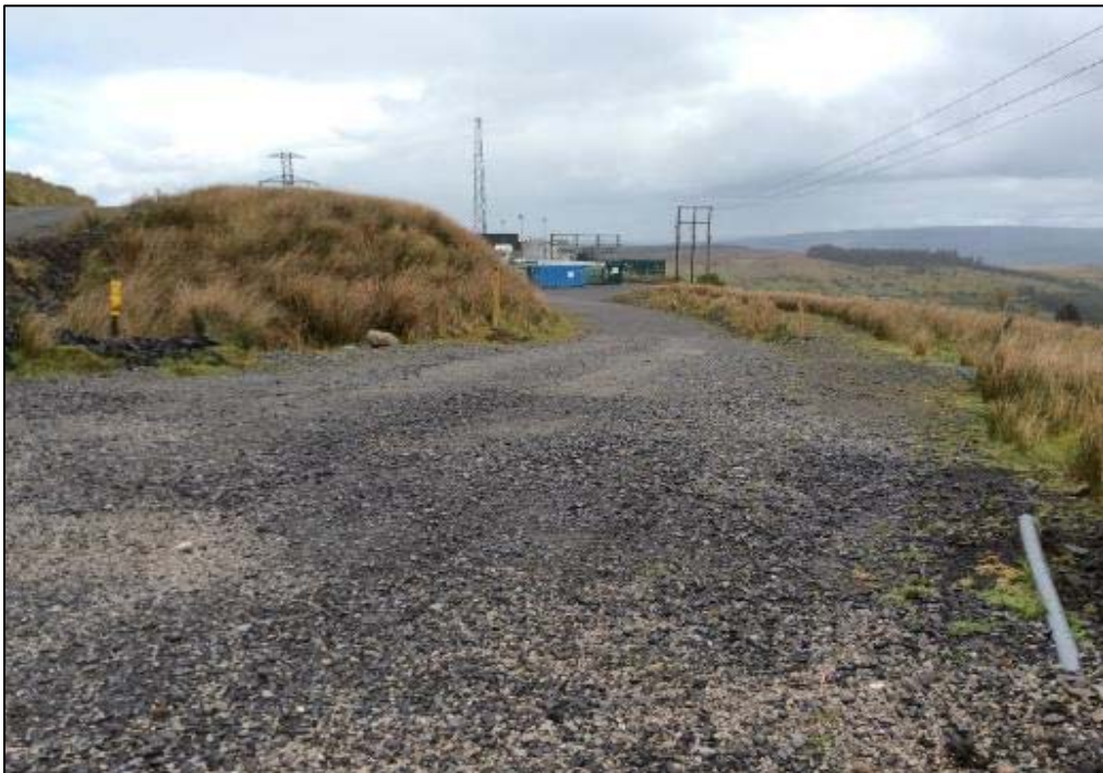
Plate 13-48 Existing Garvagh substation looking north
