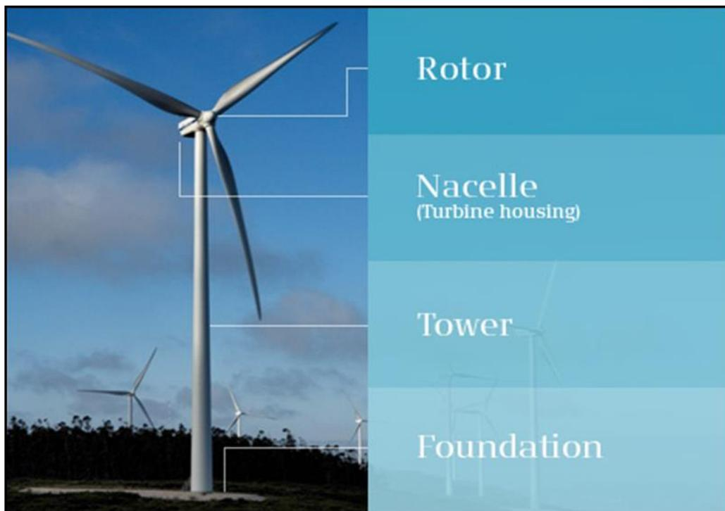
Plate 2-1 Wind turbine components
