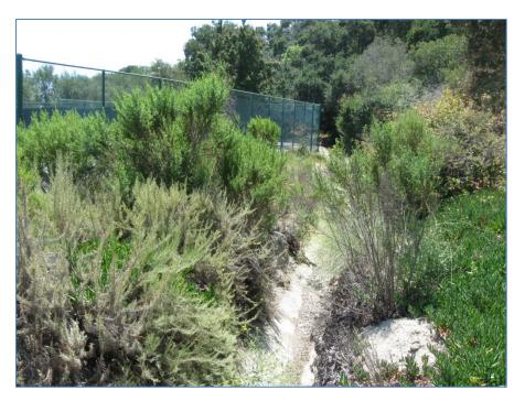
Photo 20. Concrete ditch along the Avila Beach Golf Resort tennis courts, facing south. The ditch conveys flow from the roadside drainage ditch which empties into the mouth of San Luis Obispo Creek just downstream of this location.
