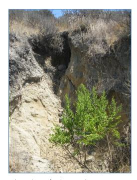
**Photo 10.** Erosional feature downslope of Culvert 3 where it connects with the gully, facing east.
