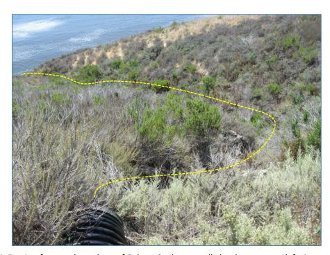
**Photo 4.** Erosion feature downslope of Culvert 2 where a gully has been created, facing southwest.
