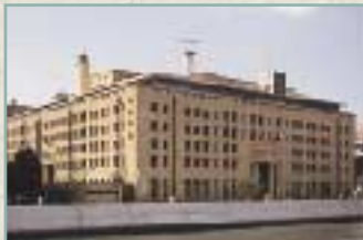
Former Sumitomo Bank's headquarters
