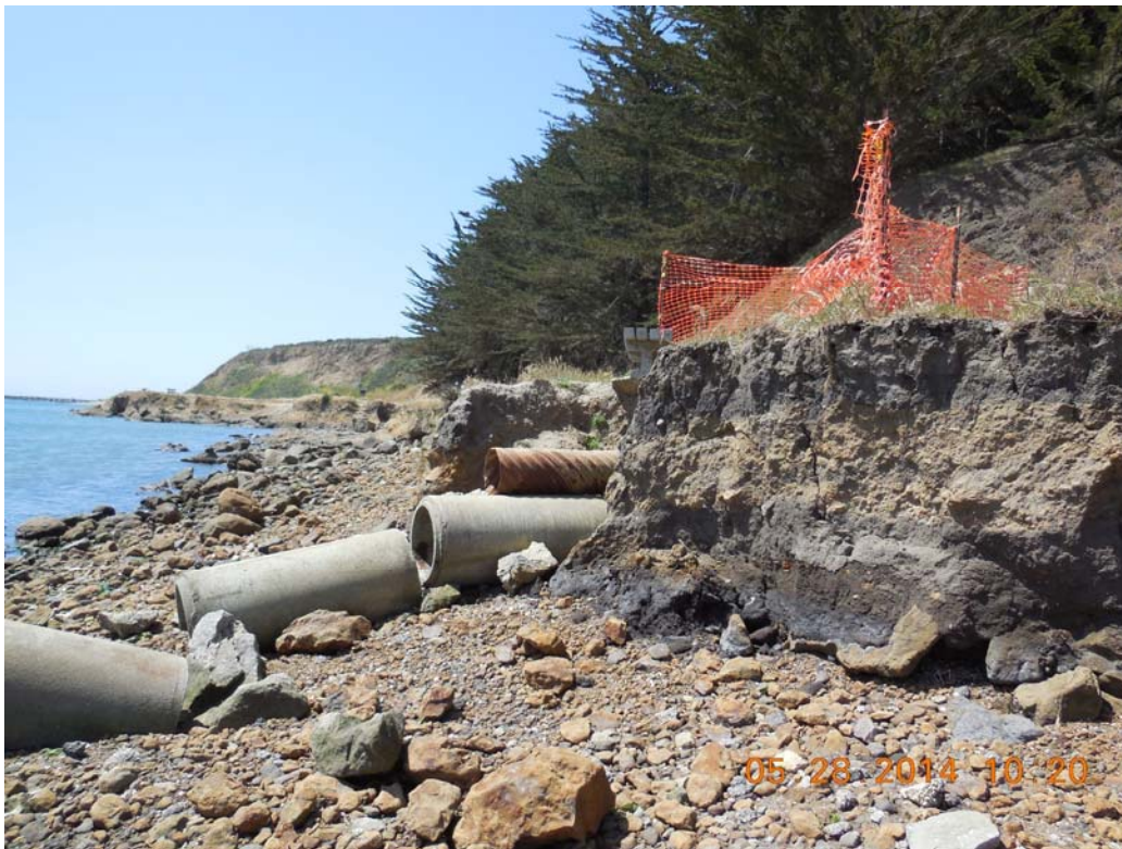
Figure 3: Culvert on harbor side.
