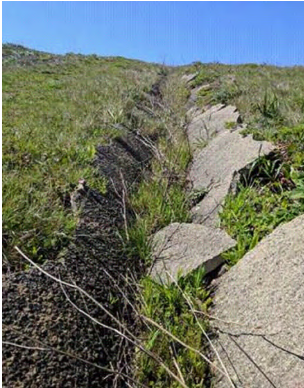
Existing Gunite Swale
