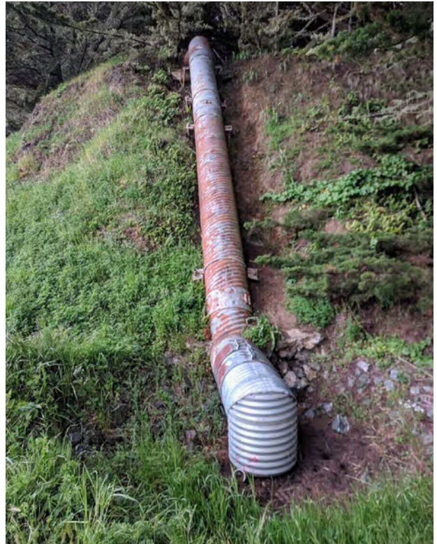
Existing Corrugated Metal Pipe
