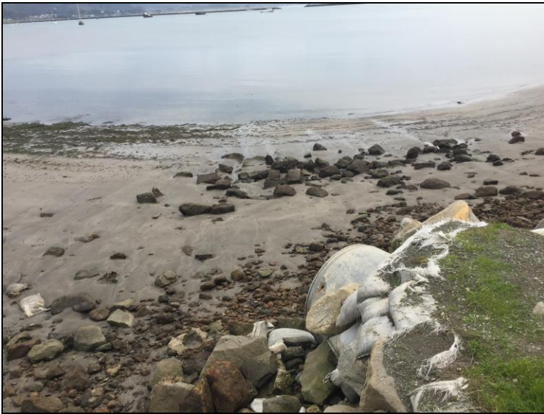
Photo 4: Tidal waters and culvert repair area.
