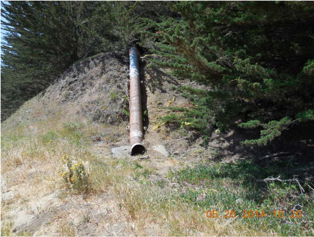
Figure 4: Culvert coming down from hillside.
