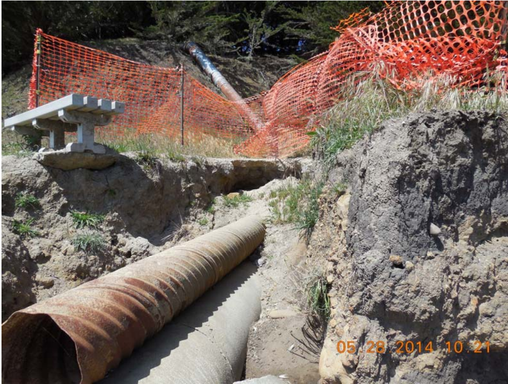
Figure 2: Looking at culvert.
