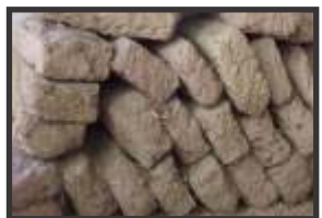
Stacked adobes from the Garcia House courtyard
