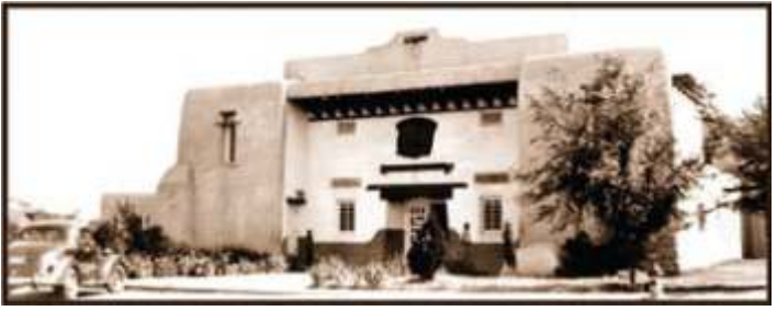
(15b) The Socorro County Courthouse is a Spanish/Pueblo Revival style building that was constructed in 1940. It has projecting vigas and wood lintels. ( photo circa 1940 )
