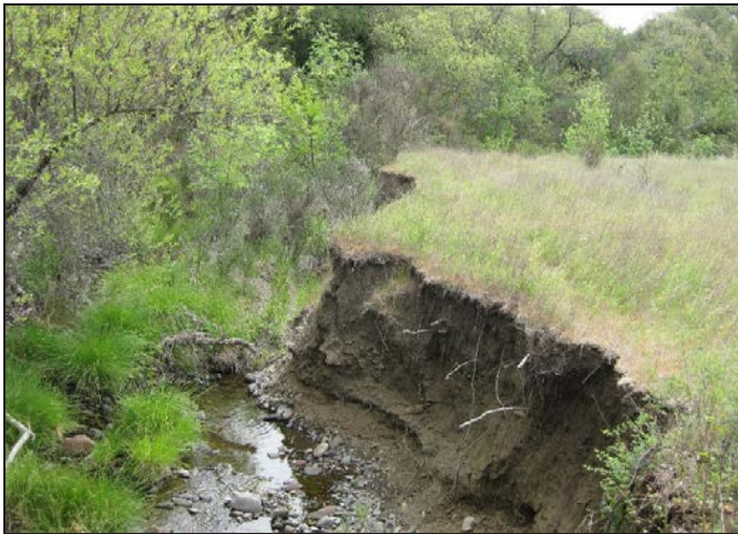
Photo 7. Weeks Creek bank erosion
