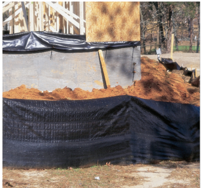
Photo 29: Silt fencing can be used as an exclusionary fencing option to prevent bullfrogs from entering in native amphibian habitat.
