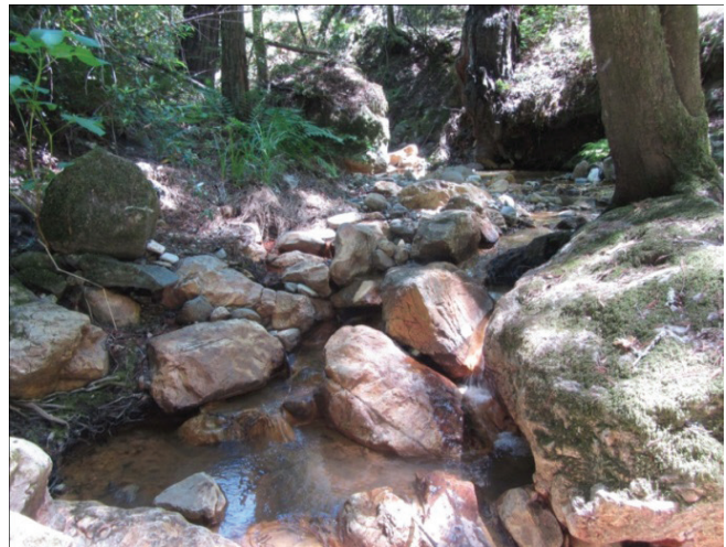
Photo 28: Calabazas Creek conditions demonstrating high percentage of large boulders indicating high velocity rain events capable of moving significant material.
