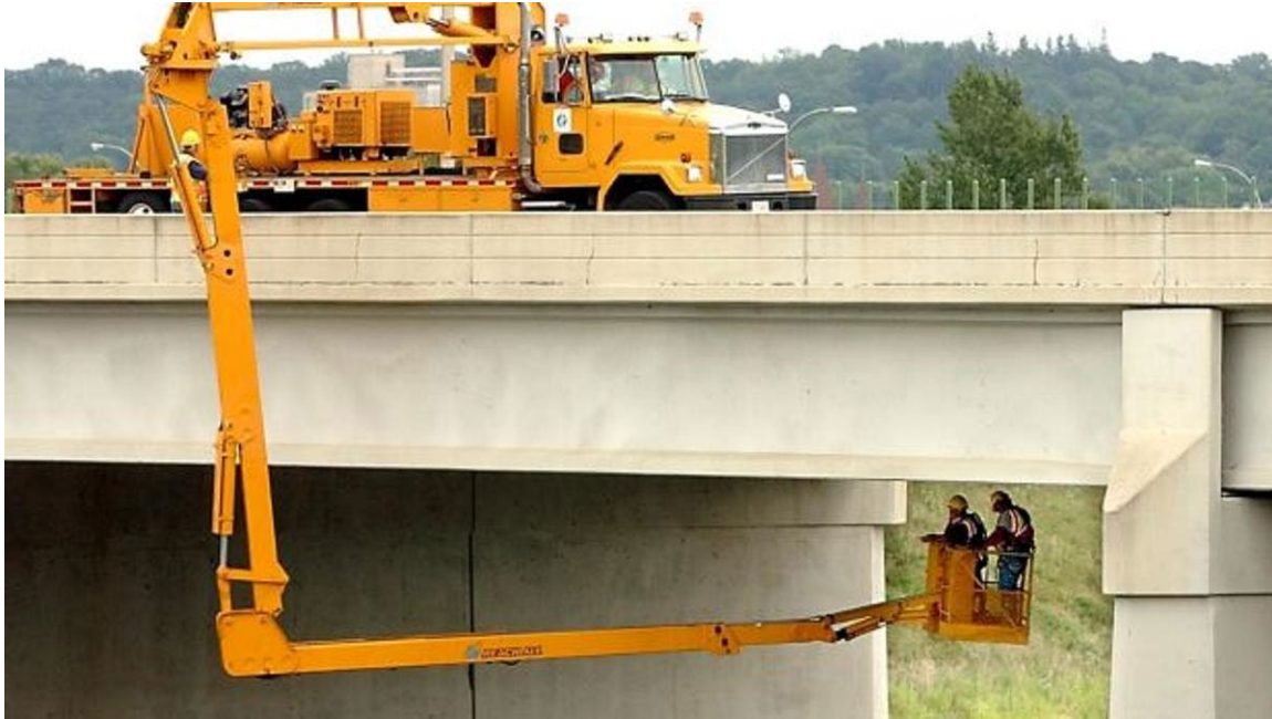
Figure 11. Example of boom truck on a bridge.
