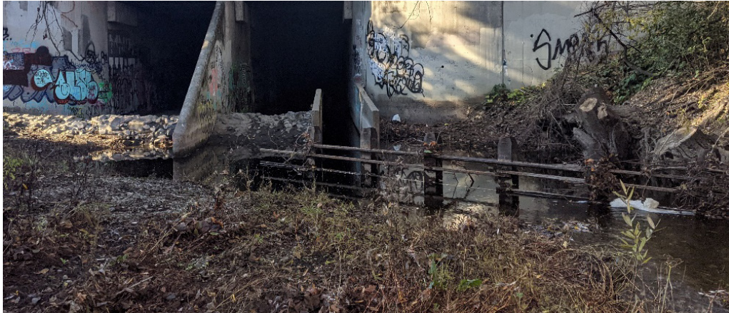
Photograph 2.2-5. Existing E Street Bridge Fishway Extension Trash Rack.
