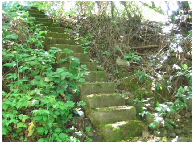
Detail of Concrete Steps
