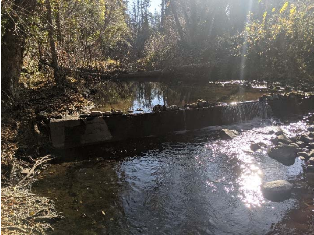
Melita Diversion Dam, Looking Southeast
