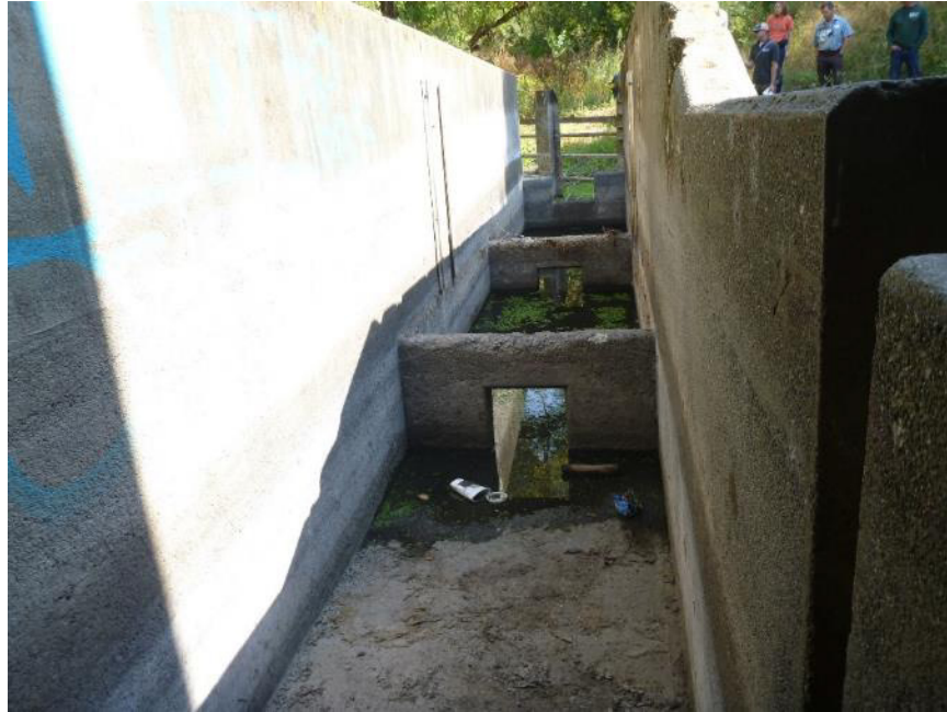
Photograph 2.2-3. Weirs Within E Street Bridge Fishway Extension, Looking Upstream.
