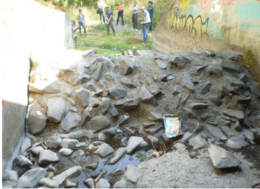
Photograph 2.2-4. Grouted Rock Weir, Looking Upstream.
