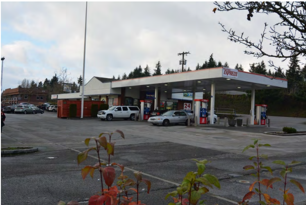
Figure 6-2 295 SW 148th Street, Burien; view to the northwest
