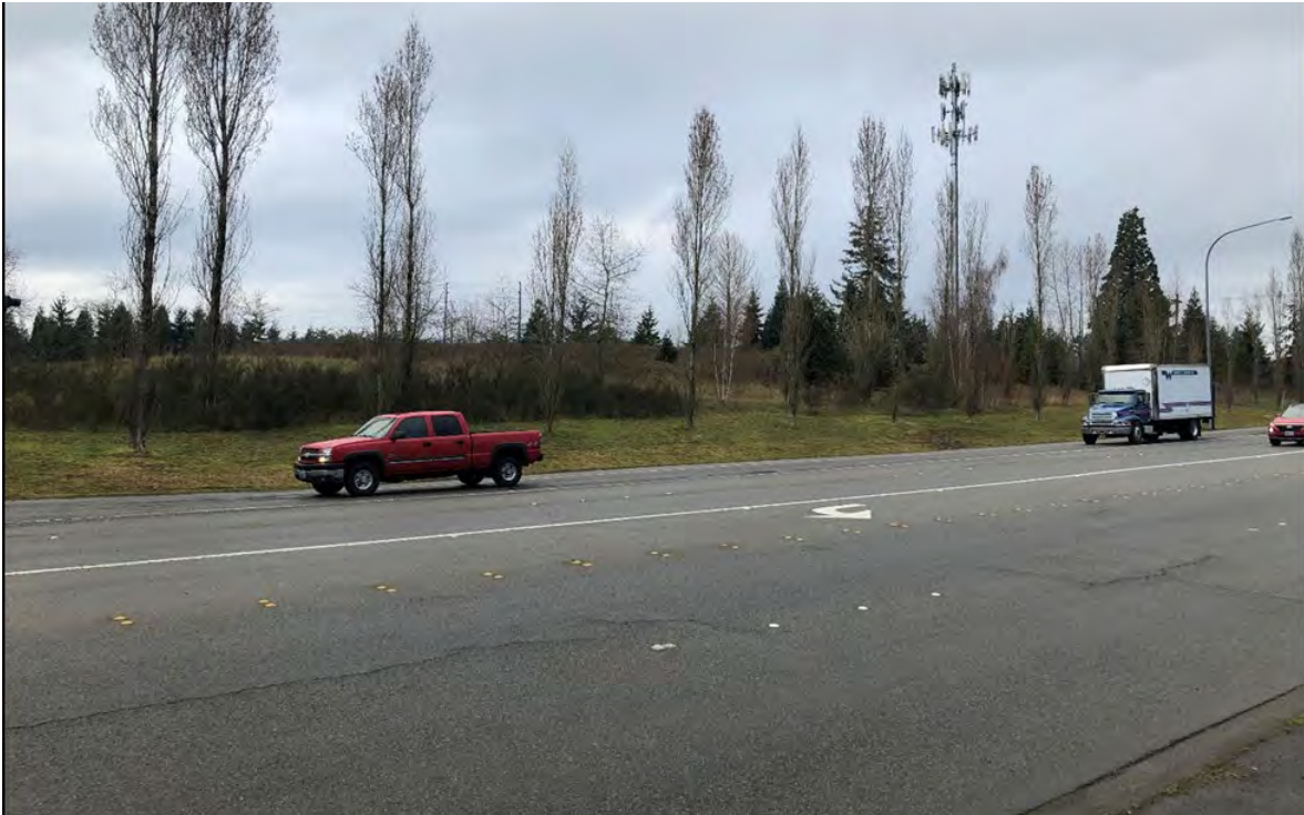
Figure 5-15 West-facing overview of the Poplar Way Interstate-5 ramp area
