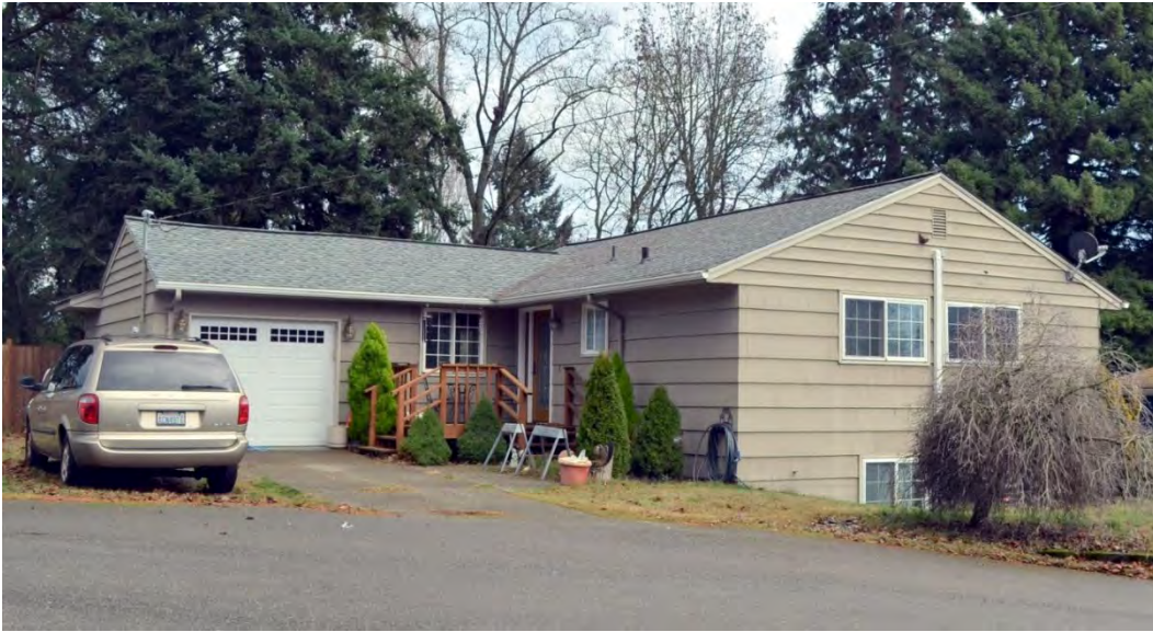
Figure 6-16 14838 5th Avenue S, Burien; view to the southeast
