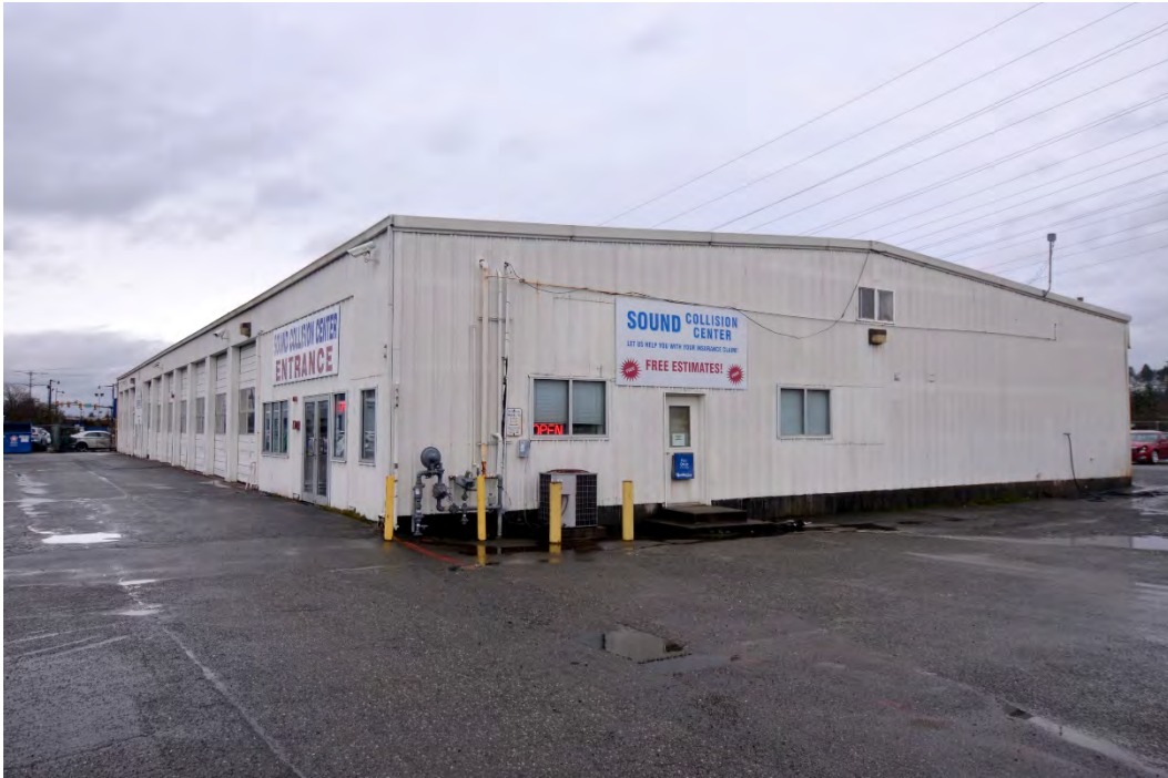
Figure 6-25 720 Rainier Avenue S – Building 2, Renton; view to the northeast
