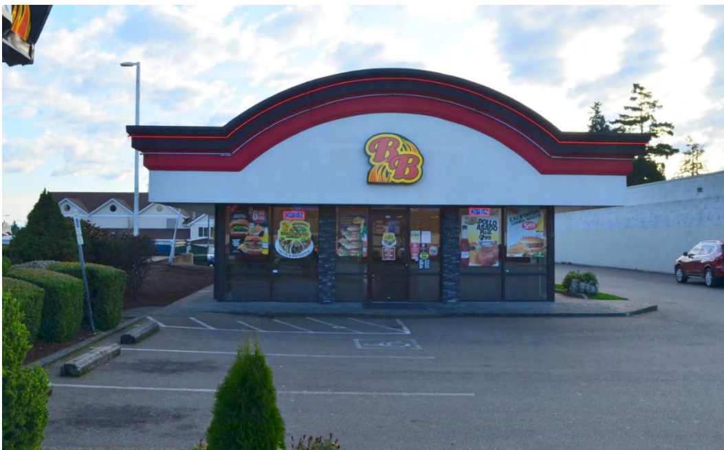
Figure 6-6 119 SW 148th Street, Burien; view to the south
