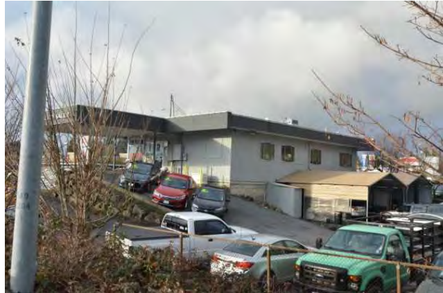
14650 1st Ave S Showroom_2019_NW.JPG
