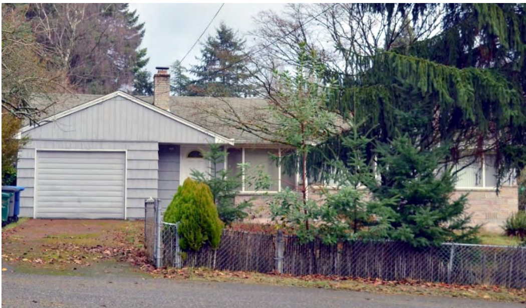
Figure 6-14 14832 4th Avenue S, Burien; view to the east
