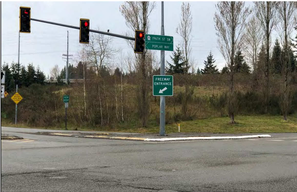
Figure 5-14 West-facing overview of the Poplar Way I-5 ramp area
