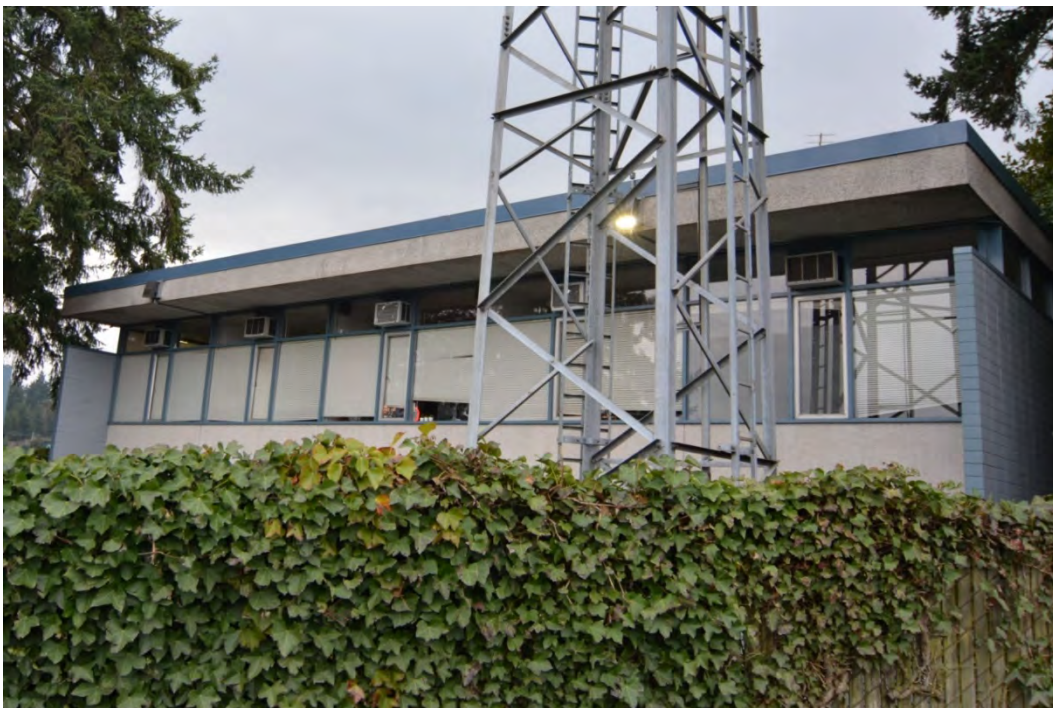
Figure 6-18 15700 International Boulevard, Tukwila; view to the southeast
