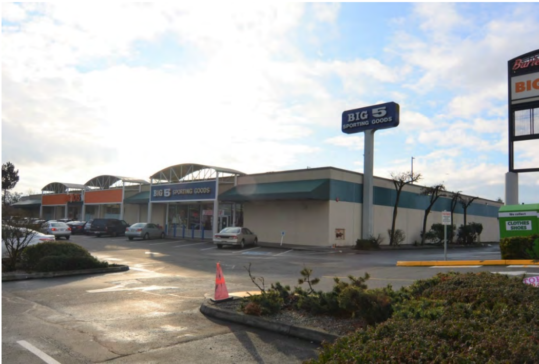
Figure 6-3 125 A SW 148th Street, Burien; view to the southwest
