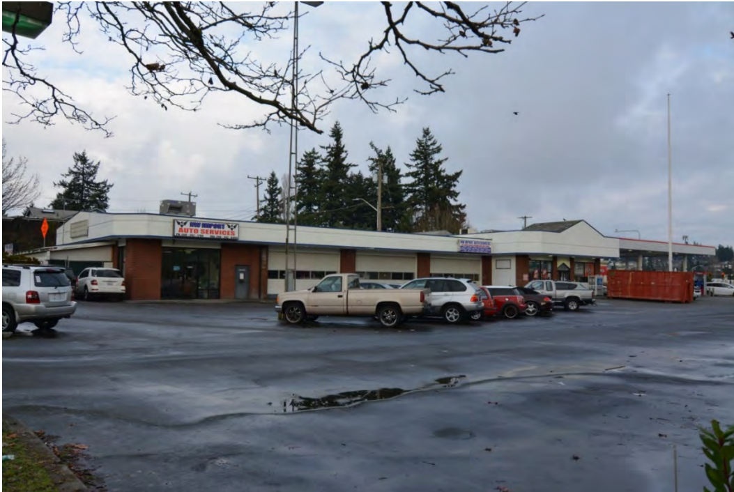
Figure 6-1 295 SW 148th Street, Burien; view to the northeast
