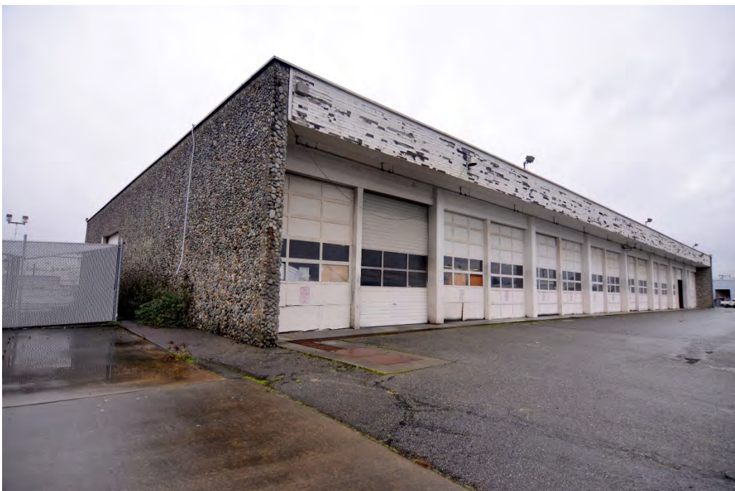
Figure 6-28 750 Rainier Avenue S, Renton; view to the view to the northwest
