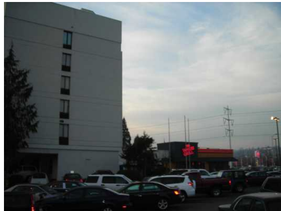
North Wing-Structure D-Far Right
