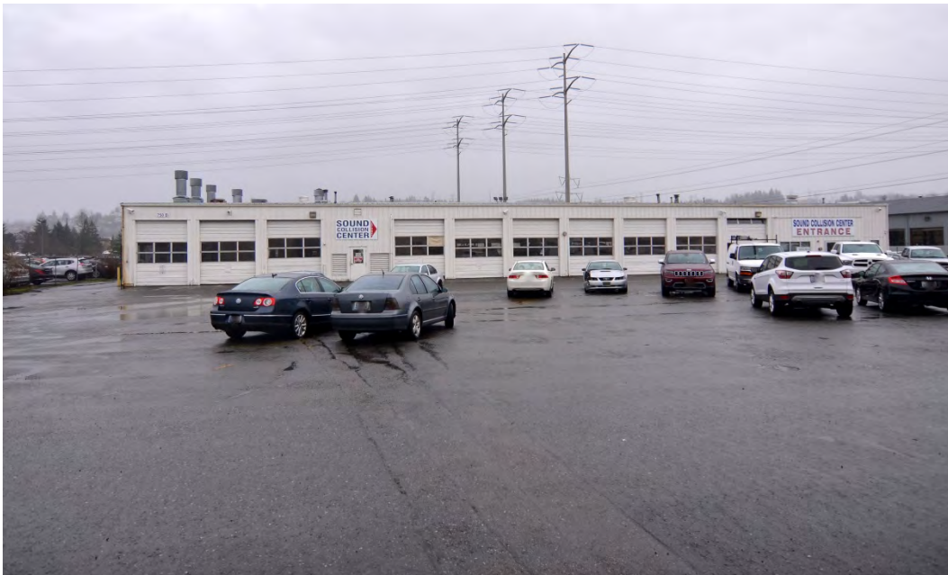
Figure 6-26 720 Rainier Avenue S – Building 2, Renton; view to the east
