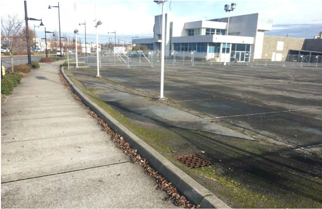
Figure 5-6 North-facing overview of the abandoned car dealership and extensively paved ground surface
