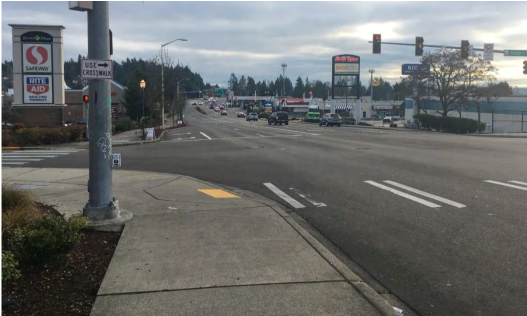
Figure 5-1 East-facing overview of north side of SW 148th Street
