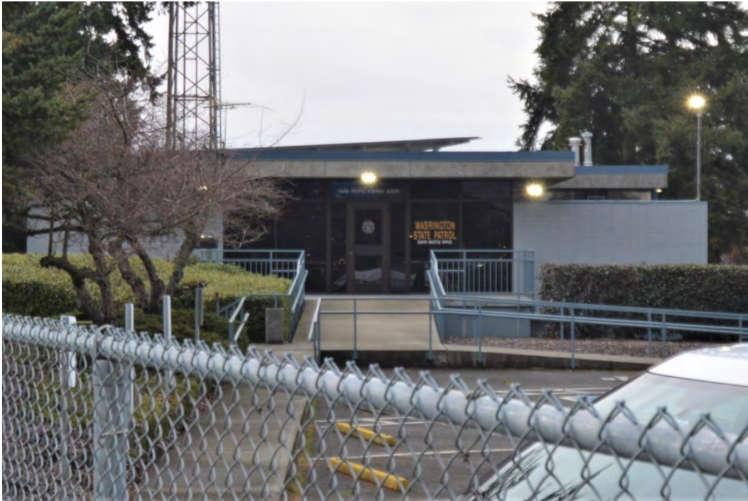
Figure 6-17 15700 International Boulevard, Tukwila; view to the northeast
