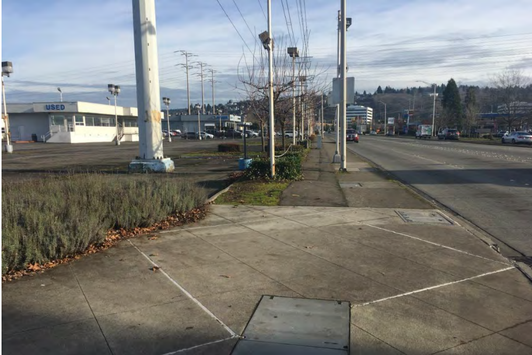
Figure 5-7 East-facing overview of the southern end of the planned South Renton Transit Center site; note multiple buried utilities, paved surfaces, aboveground power lines, and flat landform
