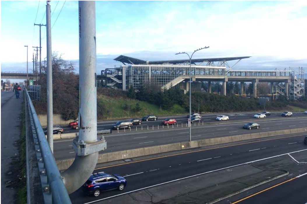
Figure 5-4 Northwest-facing overview of the SR 518 cut and Tukwila International Boulevard Station
