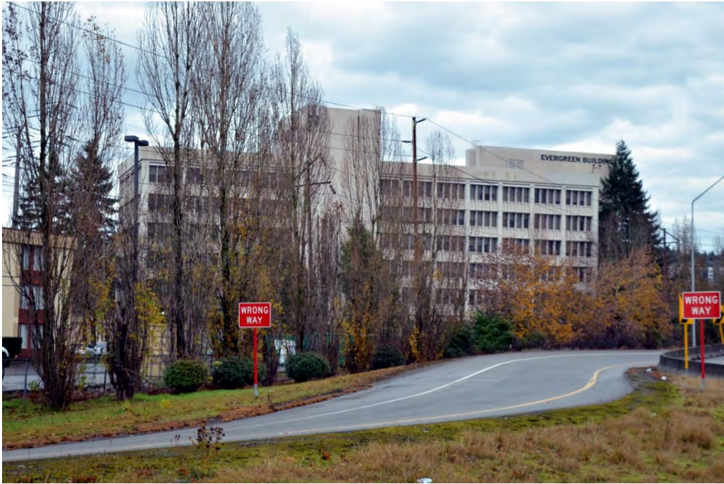
Figure 6-19 15 S Grady Way, Renton; view to the east
