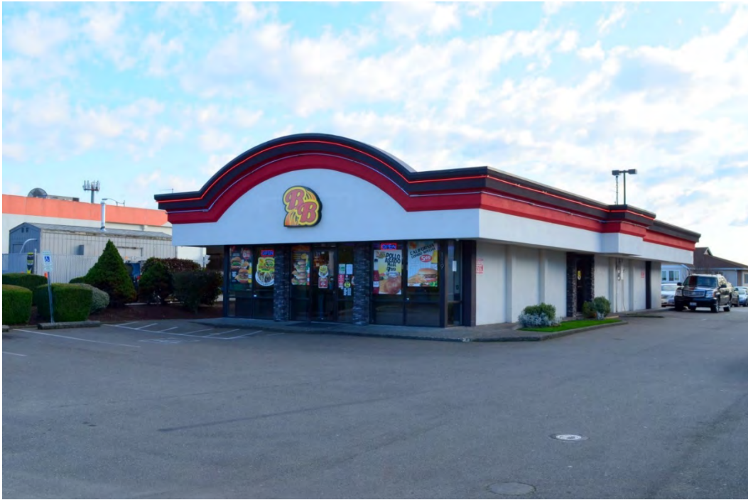
Figure 6-5 119 SW 148th Street, Burien; view to the southeast
