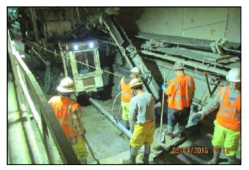
Lifting NB TBM No. I cutterhead from the UWS shaft.
