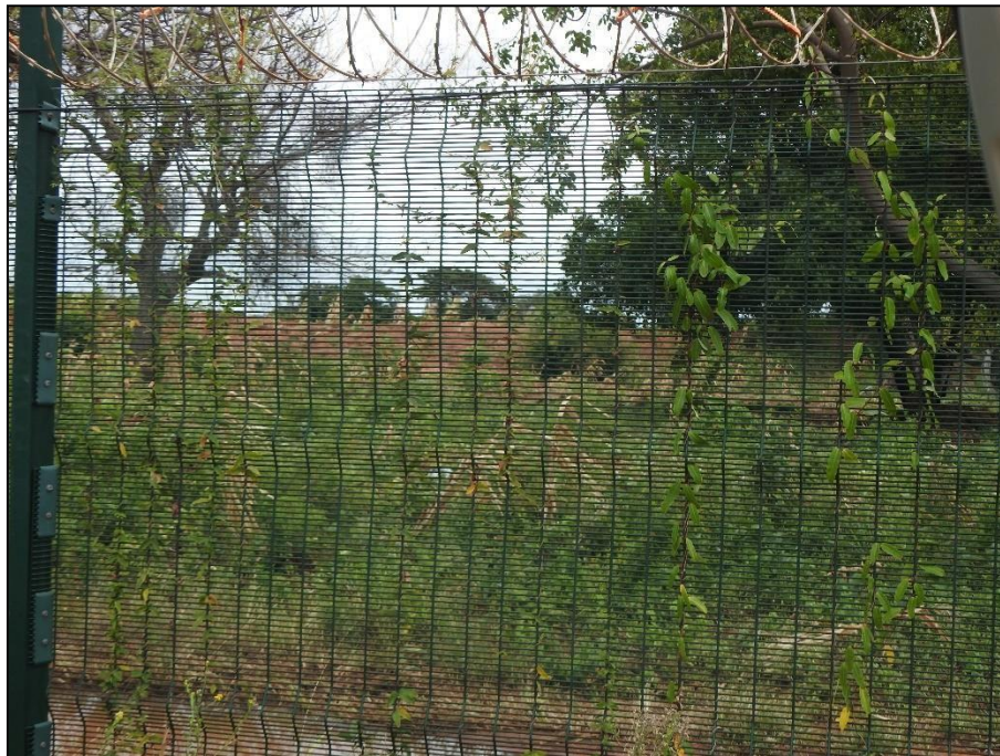
Figure 4-6 Example of the type of fencing employed at Mozal
