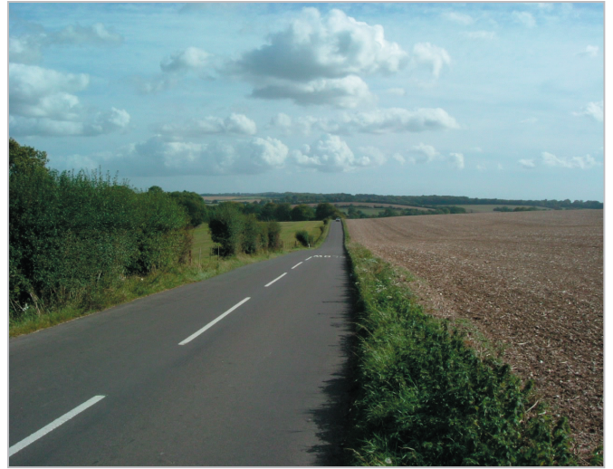
Long, straight roads cross the area.
