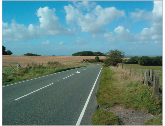
The A272 is one of the major transport routes which cross the landscape.
