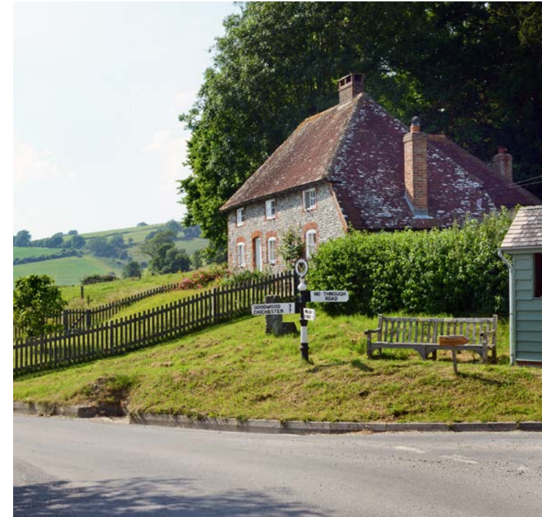
A quiet corner of East Dean village. The house walls are constructed with coursed flint, locally and plentifully available from the surrounding chalk downs.
