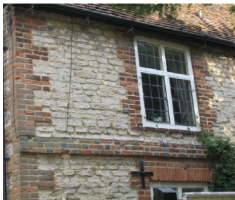
Clunch and brick at Lych Gate Cottage
