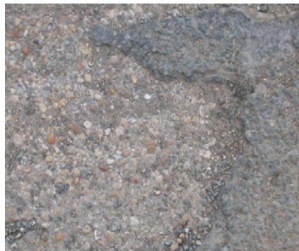
Road Surface at Bridge End
