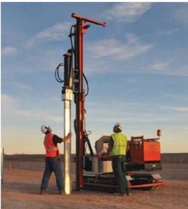
Position hydraulic ram and lift post into position beneath ram head
