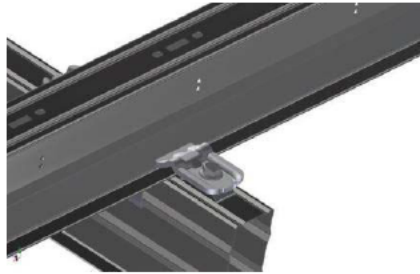
Torque purlin clamps as specified on project drawings using 16 mm socket
