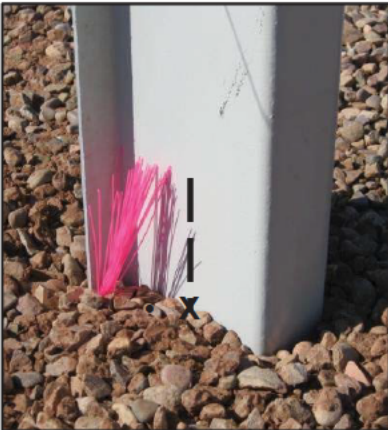
Ram two posts at opposite ends of array for string line
