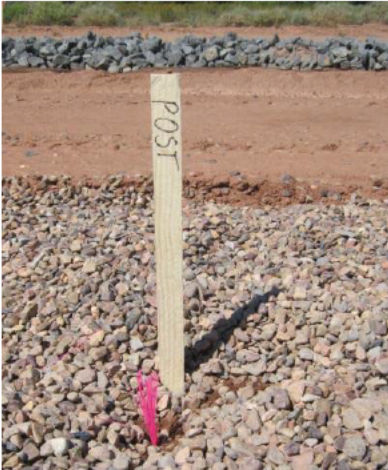
Mark each post location using soil nails with flagging
