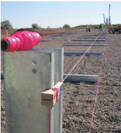
Use string line as guide to determine correct placement and depth of posts
