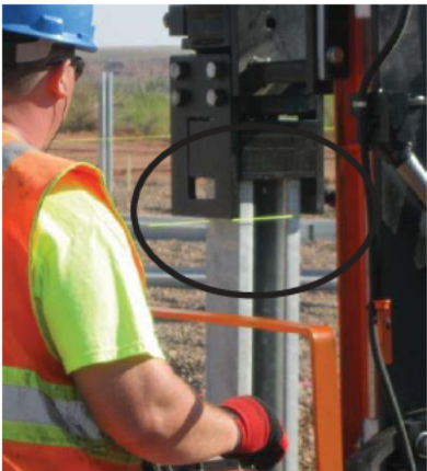
Hammer head touching top string line indicates correct depth is reached
