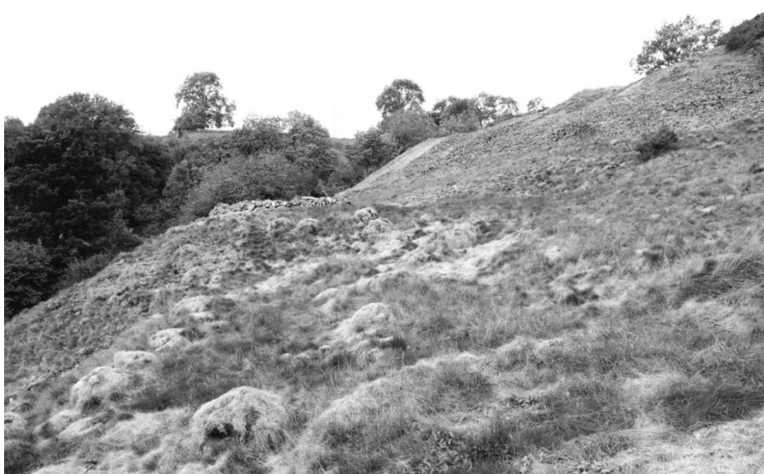
Plate 20: The dressing area next to the Footway Shaft that lies behind (Feature L); the large hillock of the main engine shaft covers a large part of the slope above (Feature H).
