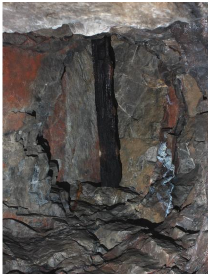
Plate 44: looking up at the surviving timber in the roof cavity at the eastern end of the hydraulic water pressure engine chamber (Photograph: Mat and Niki Adlam Stiles).
