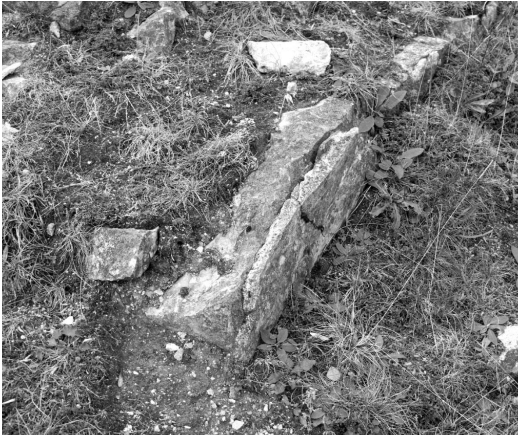
Plate 18: The ‘ore bin’ tanks had rendered sides and intact in-situ fragments of this are still visible (Feature J).
