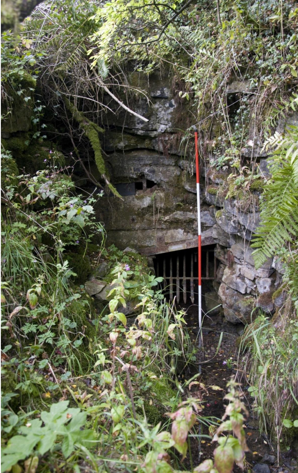
Plate 25: The partially walled-up entrance to the Dale Mine pumpway (Feature R).
