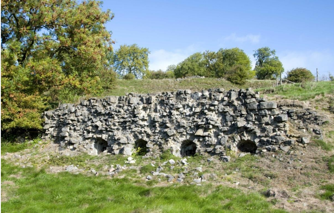
Plate 46: The south-eastern part of the ‘ore bins’, with robbed retaining wall and four openings that led from the tanks behind; the western half of the ‘ore bins’, where there were two openings, is shrouded by trees but with one of these just visible.
