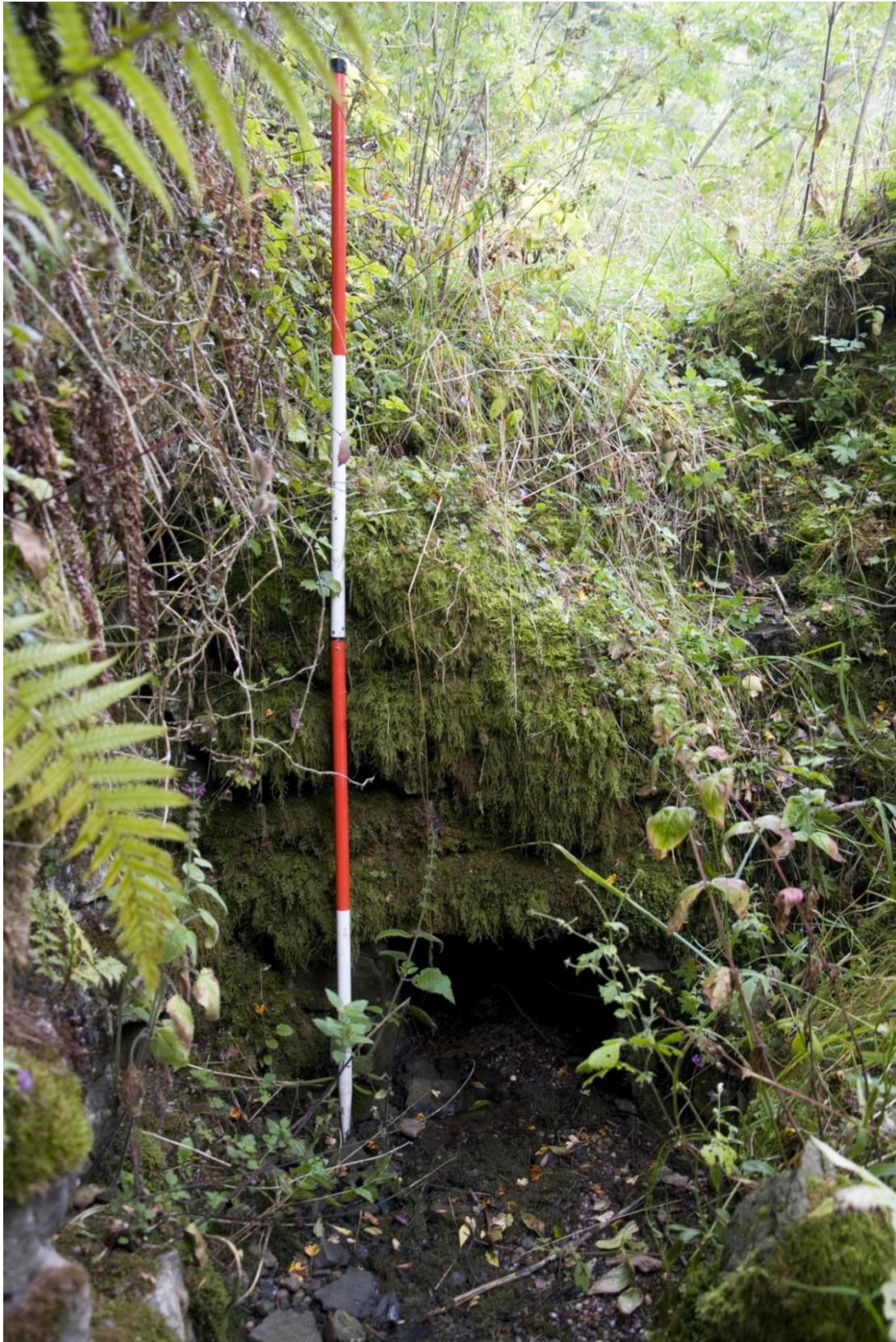
Plate 26: The covered bolt that takes the water from the Dale Mine pumpway to the river (Feature R).
