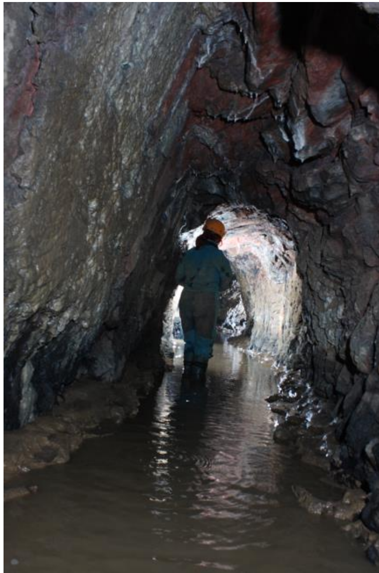
Plate 30: In the pumpway level, near its start, with left wall at a hading fault (Photograph: Mat and Niki Adlam Stiles).
