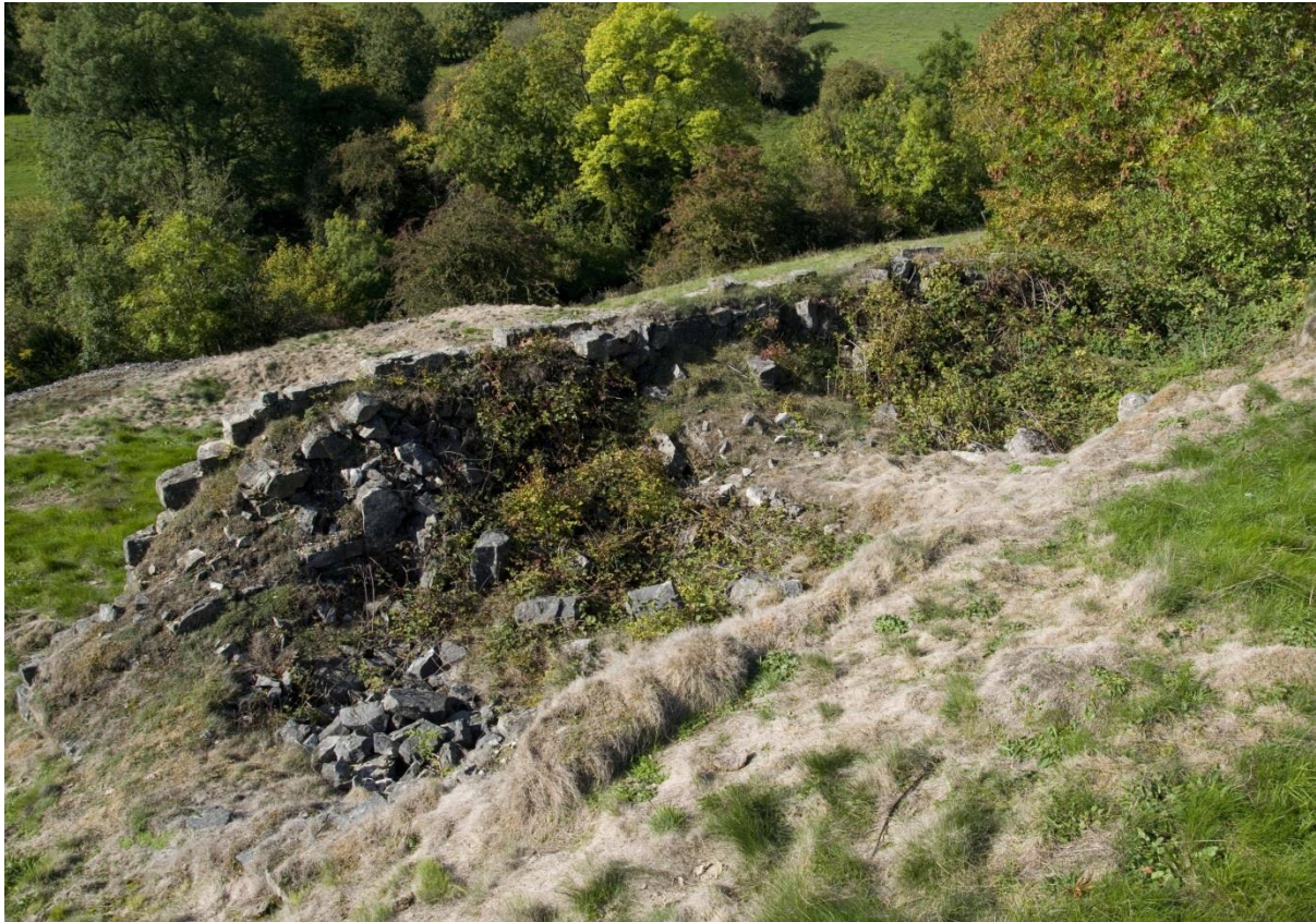
Plate 12: The south-eastern end of the ruined bank of ‘ore bins’ (Feature J), with rubble-choked tanks visible.
