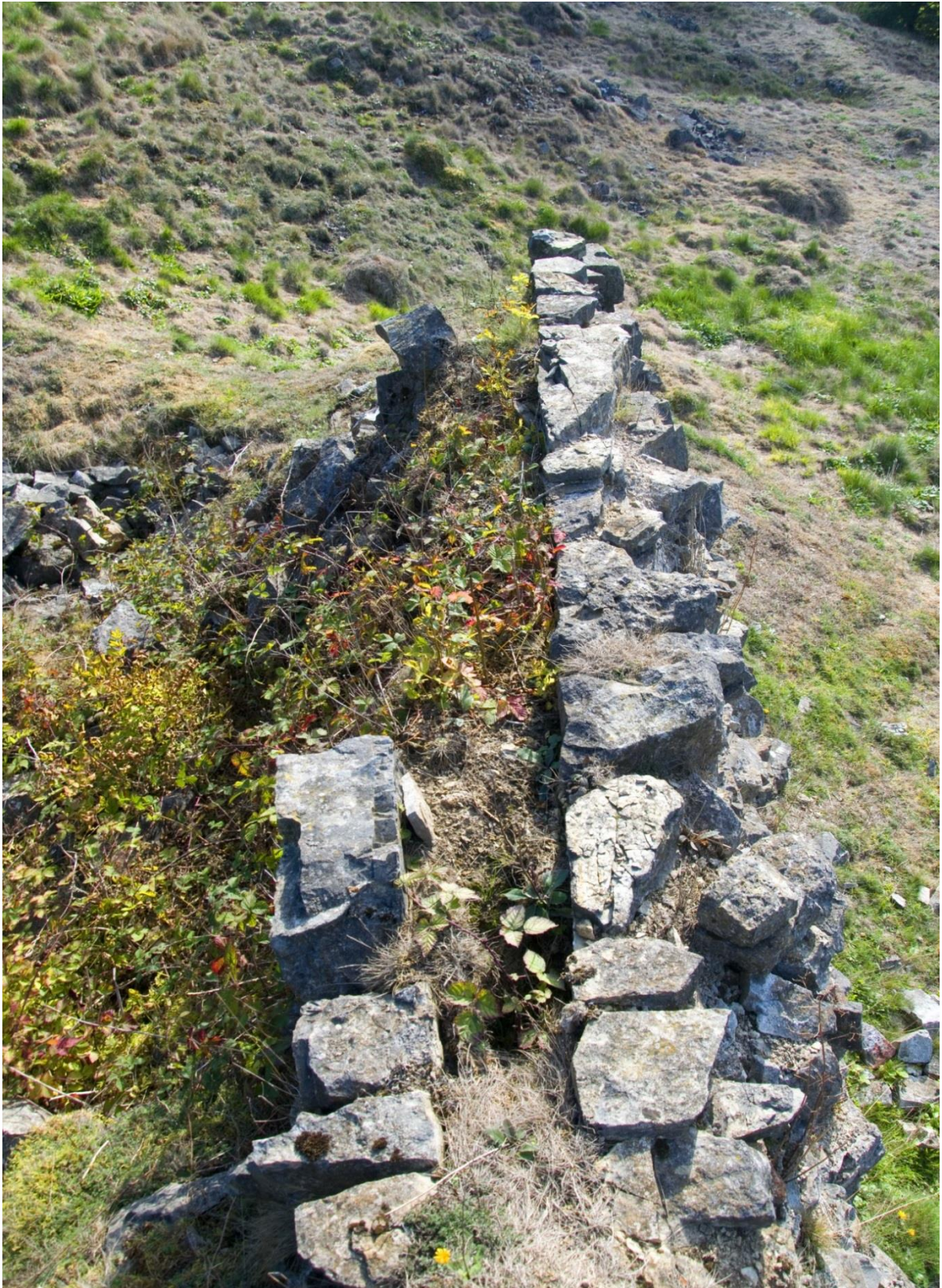
Plate 14: The top of the retaining wall of the south-eastern ‘ore bins’, showing the two adjacent wall faces with a gap between that matches the position of the long lintel at the timber frames in the openings below; the other faces of the two walls have been robbed in both cases (Feature J).
