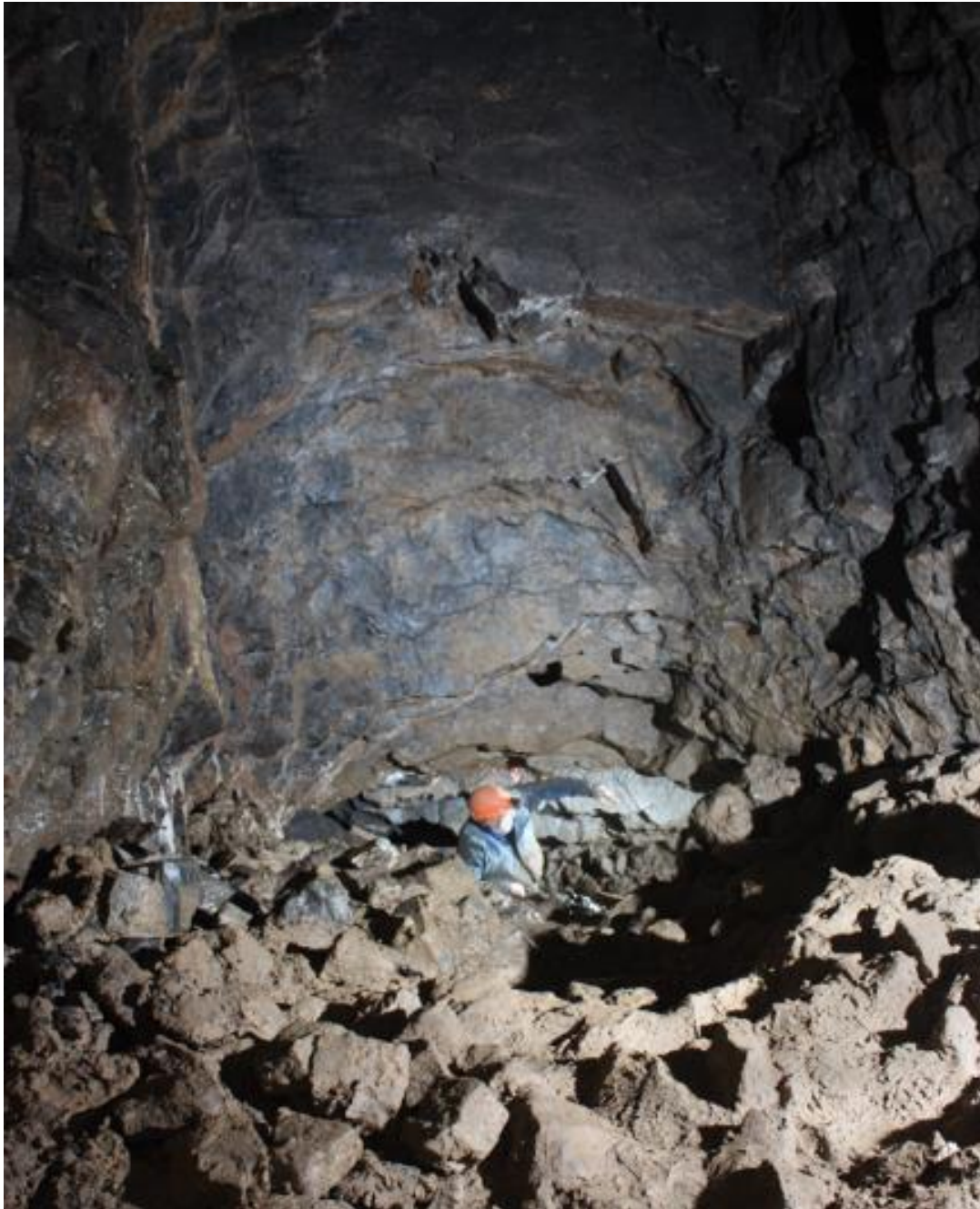
Plate 35: The south-western end of the abandoned engine chamber, part backfilled with deads, with the pumpway extension out of clear sight below the figure climbing up (Photograph: Mat and Niki Adlam Stiles).
