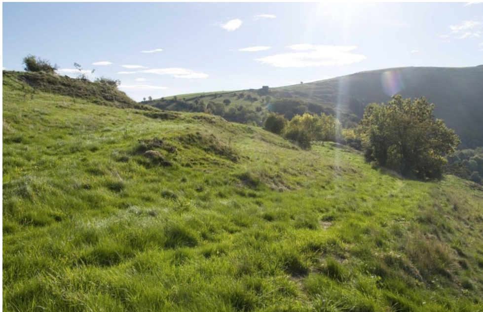
Plate 28: The main access roadway used in the late phases of mining (Feature W), leading diagonally downslope to the engine shaft area to the right, with a lower branch down to the lower dressing floor and ‘ore bins’ hidden by the small trees here; Ecton Hill lies behind.
