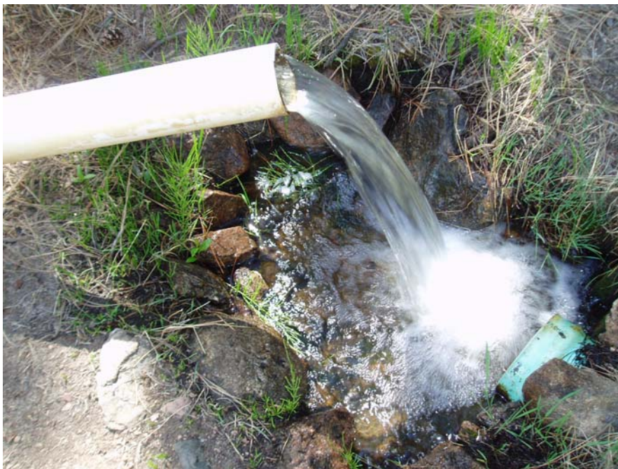
4b: Upper end of intake pipe, releasing water into ditch.
