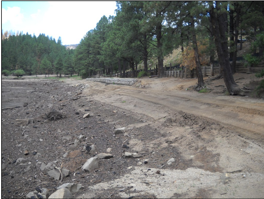
Figure 6. Access route along the east shore of Bonito Lake showing rock-filled gabion baskets for shoreline bank protection, railroad-ties for hill slope protective works, and two roadside rainwater drainage culverts, upper right. View approximately to NW. Photograph No. 4649; 7-30-2012.
