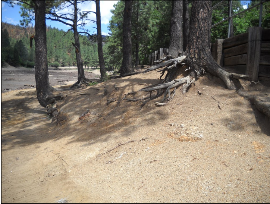
Figure 8. Photograph showing effects of wave action erosion and railroad-tie bank stabilization with hand-railing for public access to the Bonito Lake shoreline. View approximately to NW. Photograph No. 4634; 7-30-2012.
