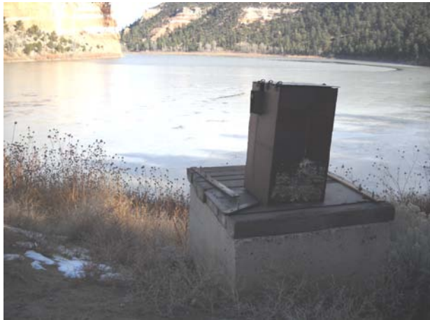
a. Acequia intake structure on dam and reservoir
