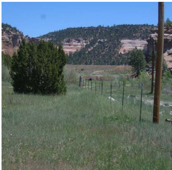
c. North pipeline re-route along fence
