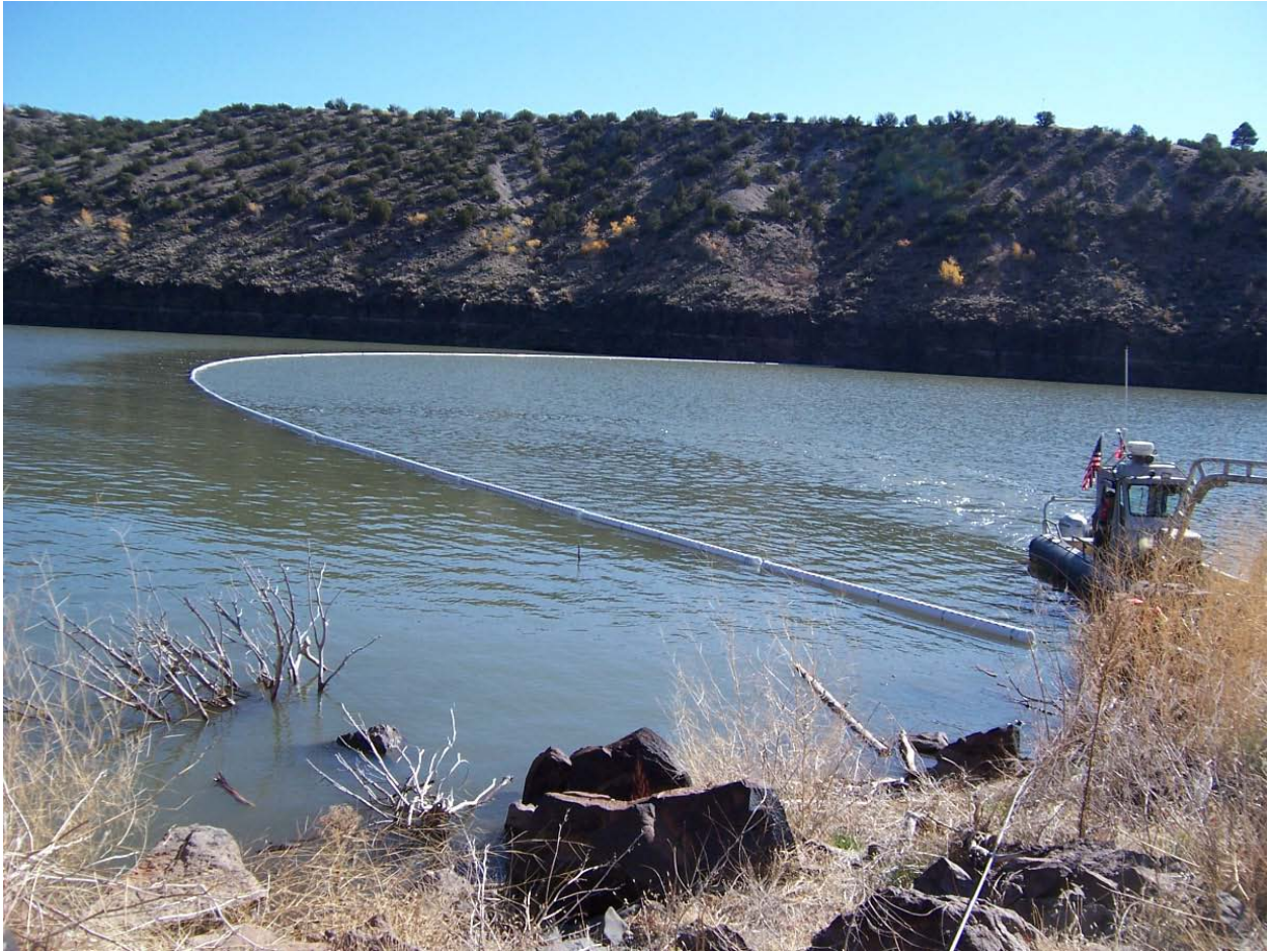
a. Boom has been towed to site, ready to anchor to banks
