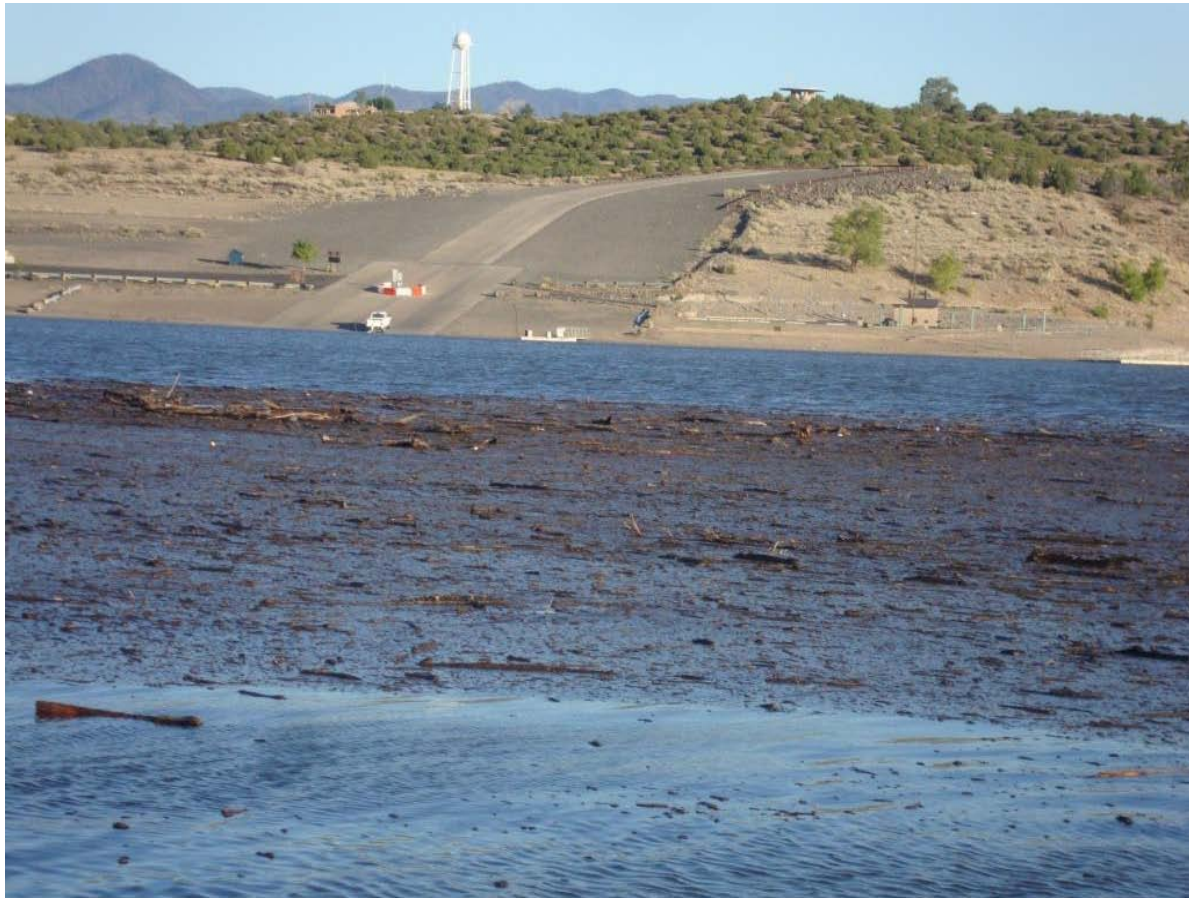
a. Floating debris obstructing Tetilla Peak boat ramp
