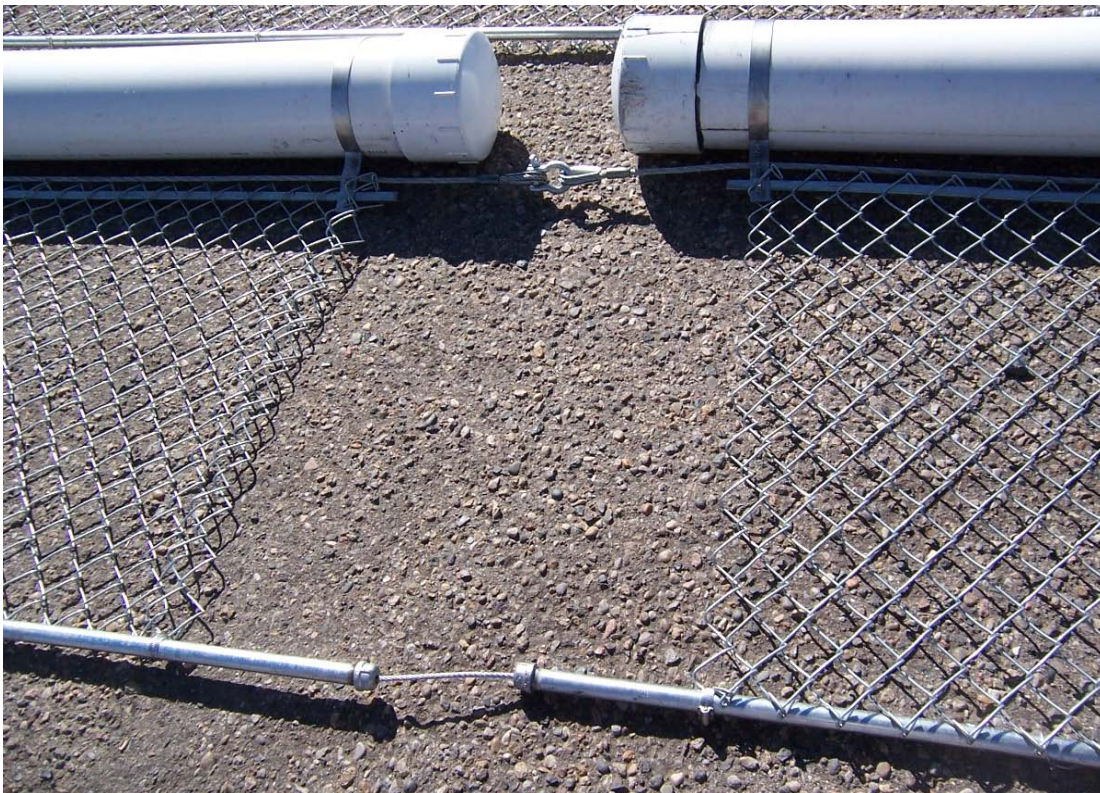
b. Connection between boom sections.
