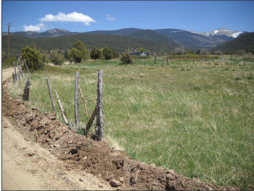
Figure 4.7. Staging Area 2, facing southeast.
