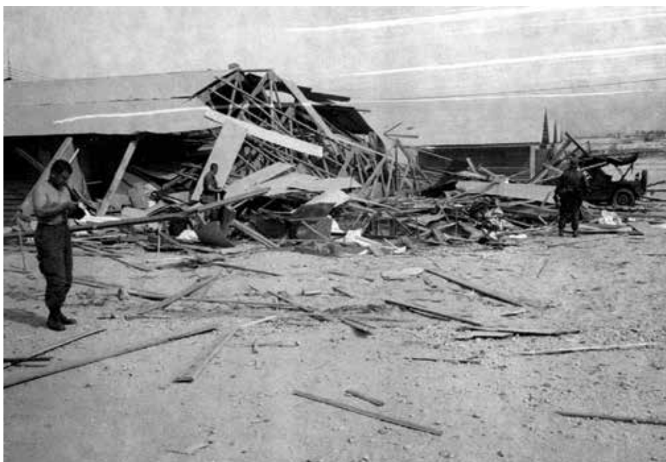
Damage at FOB 4 after the attack.
