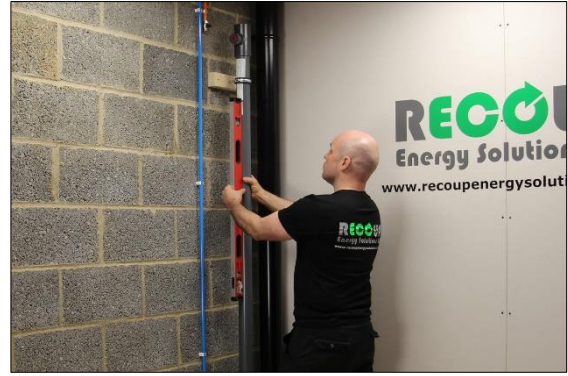
14. Check the pipe has been installed vertically and within a tolerance of +/- 20mm. Once the position is confirmed fully tighten the clamps
