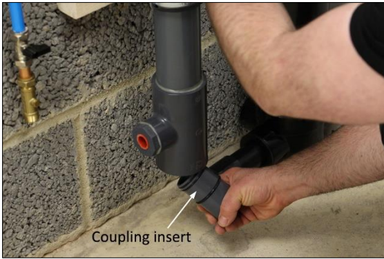
31. Push a coupling insert (Item 2) into the bottom of the Pipe+ HE.
