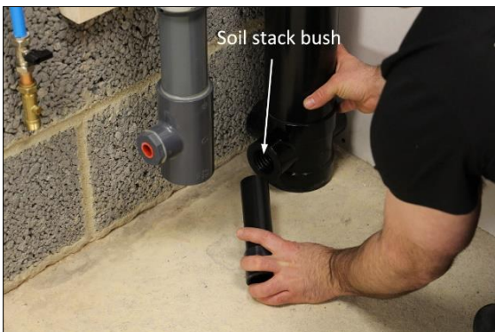
29. Insert the opposite end of the 43mm solvent weld pipe into the rubber bush of the soil stack junction.
