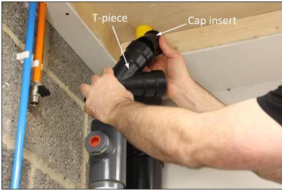
19. Push the Cap insert (Item 4) into the top of the straight section of the T-piece (Item 3). The straight position must not be used to connect to the shower waste pipe.
