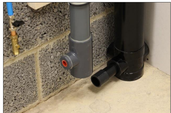
30. Push the pipe further into the soil stack than needed to assist with the connecting to the Pipe+ HE.
