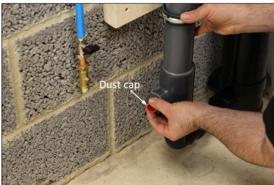
35. Remove the red dust cap from the cold water connection at the bottom of the Pipe+ HE.
