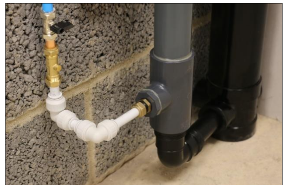
42. PVC connections could be used for connecting the mains cold water feed but copper is considered best practice.
