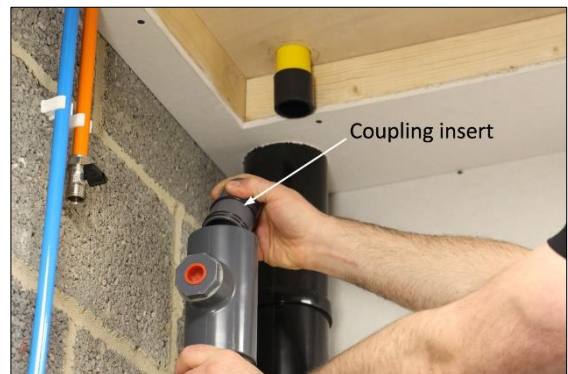
18. Push a coupling insert (Item 2) into the top of the Pipe+ HE.
