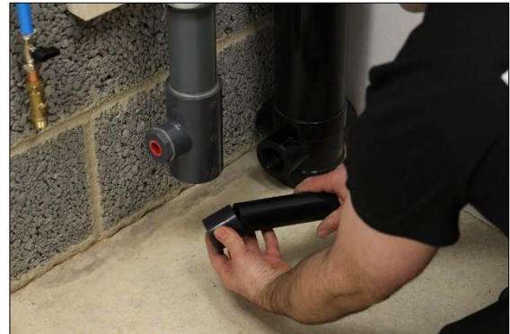
28. Push the reducer (Item 10) onto the \varnothing 43mm solvent weld pipe and allow adhesive to set.
