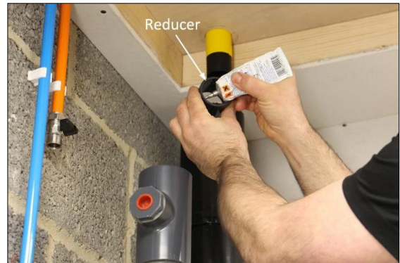
16. A \varnothing 50mm reducer (Item 10) is supplied for use with \varnothing 43mm solvent weld pipe. Apply solvent adhesive on the inside of the reducer.
