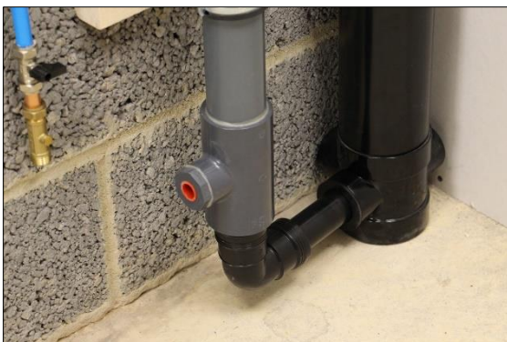
33. Slide the pipe and reducer out of the soil stack bush and connect to the open end of the 90° connector (Item 9).
