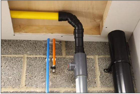
25. If the shower is located further away from the Pipe+ HE position and the shower waste pipe runs horizontally then the constructed coupling can be manipulated to allow for this.
