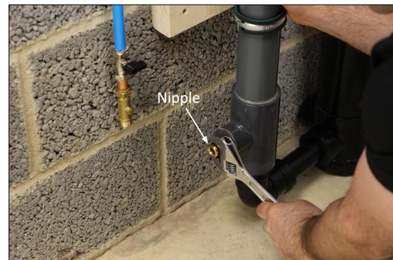
36. Connect one of the 1/2" Male BSP double sided nipples (Item 7) to the bottom of the Pipe+ HE and tighten with a spanner. Take care not to overtighten.
