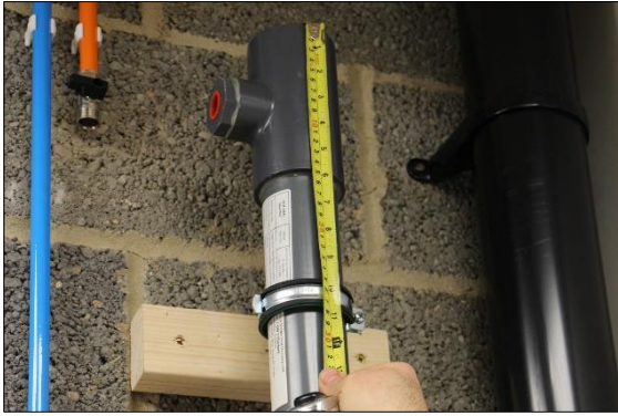
13. Check the position of the mounting brackets from the end of the Pipe+ HE and adjust if required. Should be approximately 250mm top and bottom.
