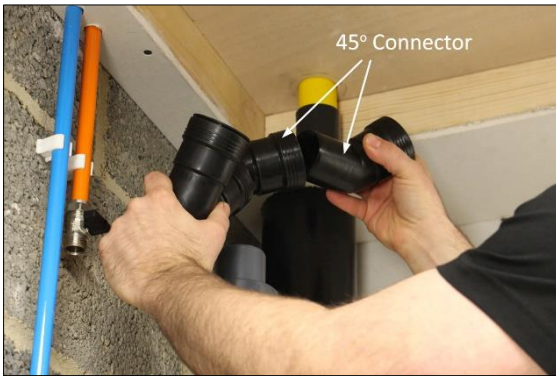
21. Insert the second 45° connector (Item 5) into the end of the other.
