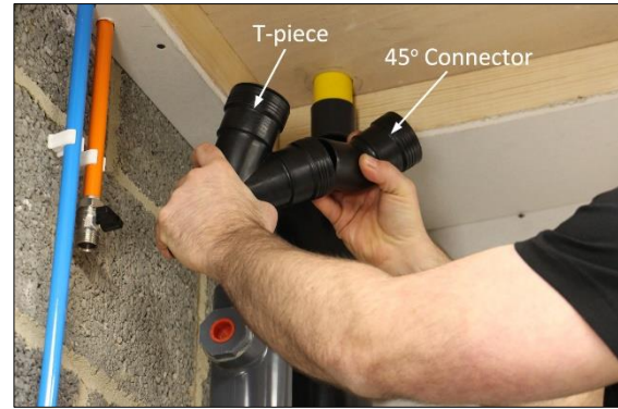
20. Insert one of the 45° connectors (Item 5) into the 45° opening of the T-piece (Item 3).
