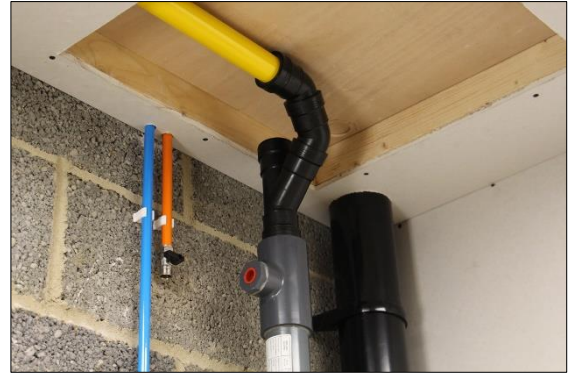
26. The constructed coupling will manipulate to multiple positions either vertical or horizontal but all components must be used in the order shown.
