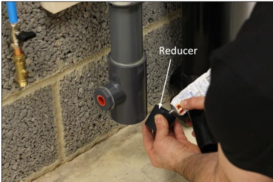
27. The soil stack connection pipe needs to be either a \varnothing 50mm push-fit or a \varnothing 43mm solvent weld pipe. A second \varnothing 50mm reducer (Item 10) is supplied to connect to a \varnothing 43mm solvent weld pipe. Apply solvent adhesive on the inside of the reducer.
