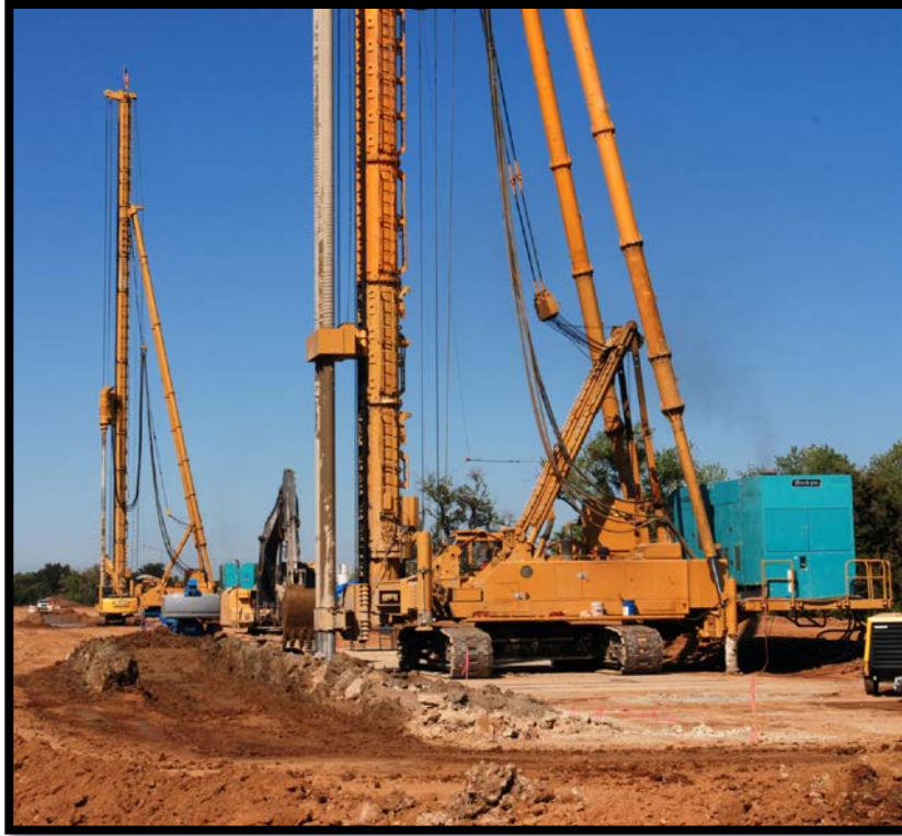
Figure 6. Slurry (Cutoff) Wall Construction Using DMM.
