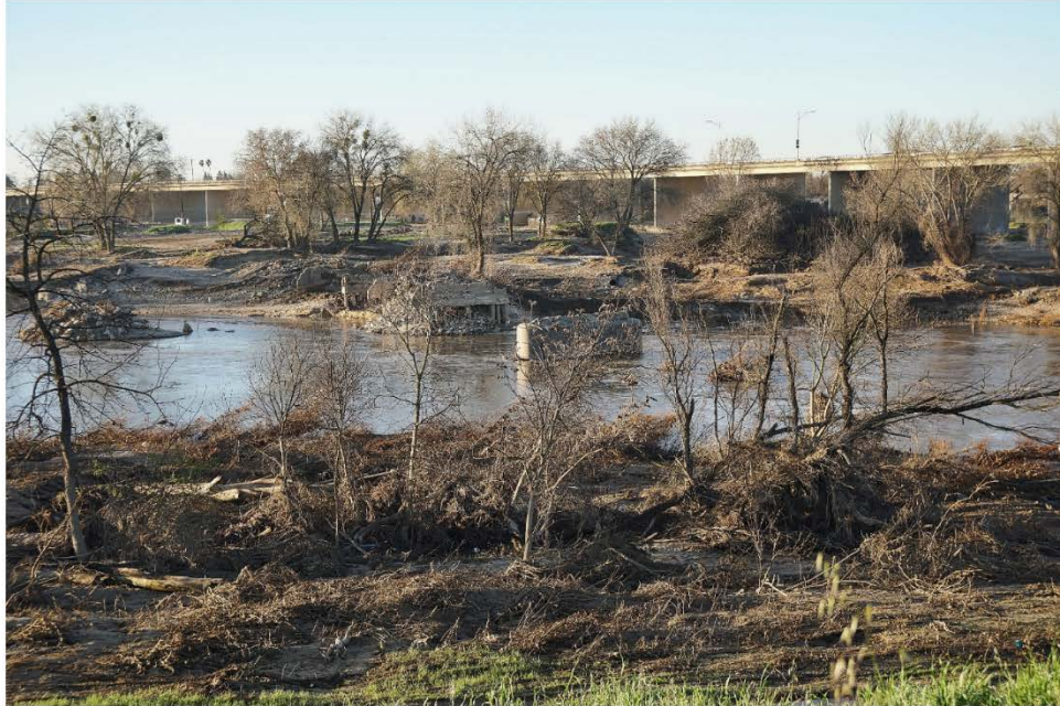
Photo 01: South side of levee after Oroville Dam release in phase 2C
