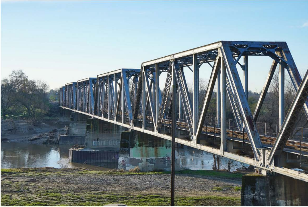
Photo 03: Railroad Bridge in phase 2A
