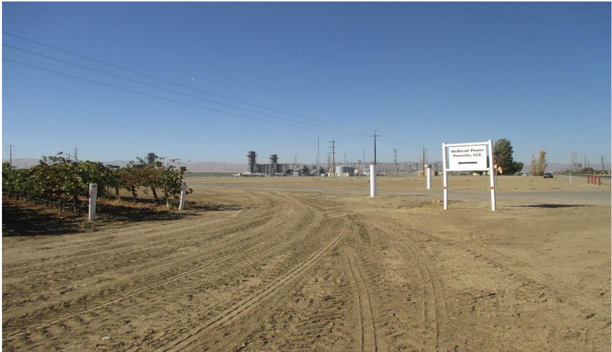
Photo 36: View of Study Area 13 facing west towards Panoche Substation.
