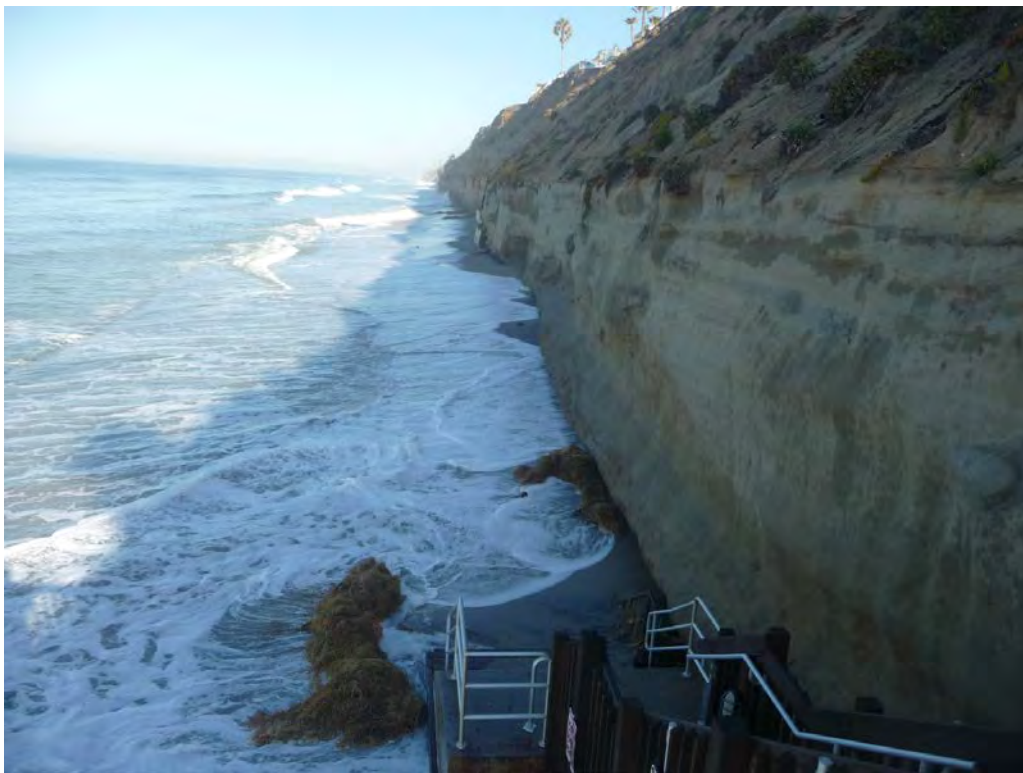
Figure 10.3-1 Wave Inundation at beach in Encinitas
