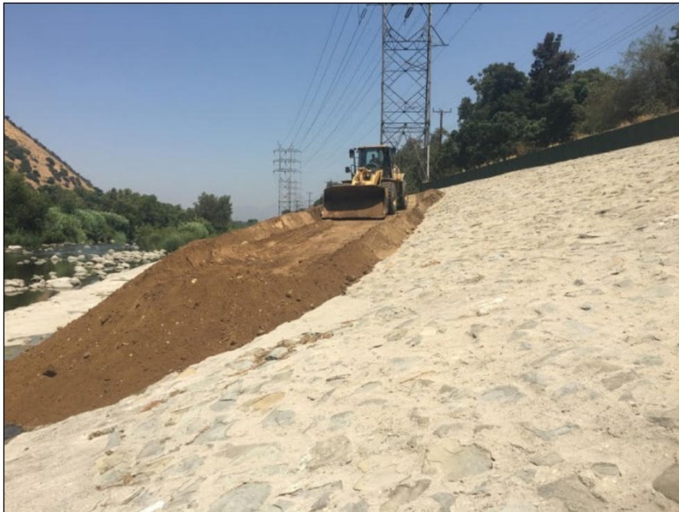
Figure 6- Example of temporary access ramp and fill placement
