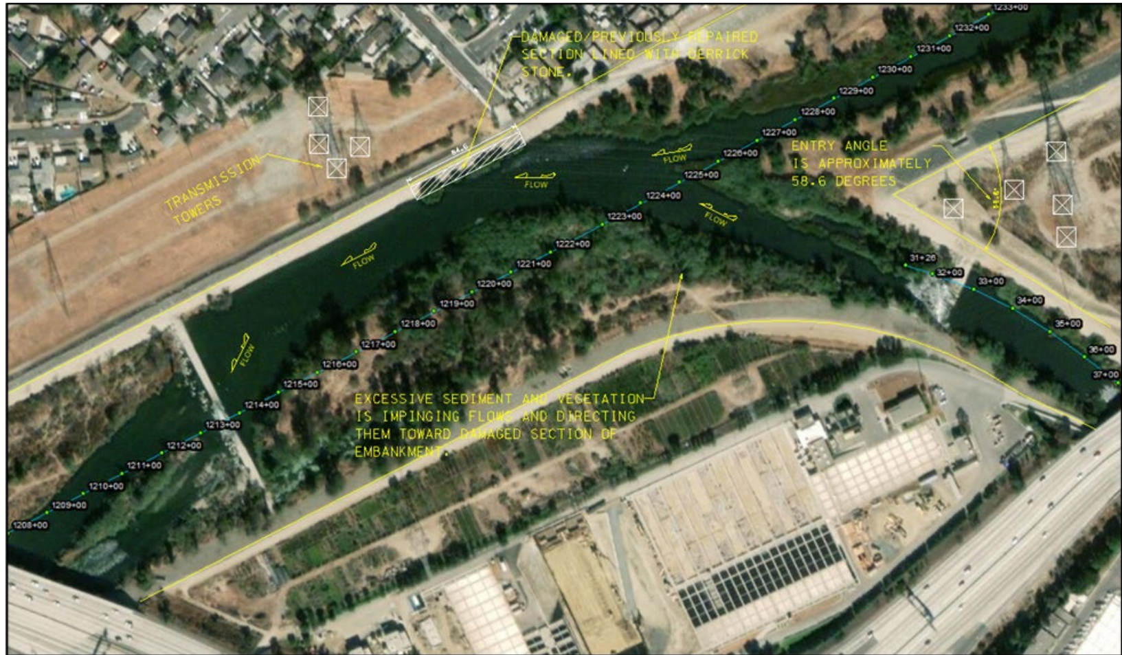
Figure 1. Excessive sediment and vegetation have directed flows at the levee's embankment
