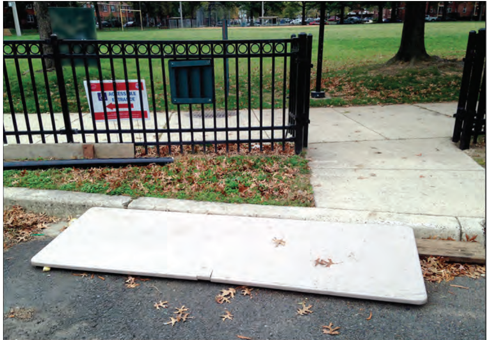
Figure 6: Example of a Polling Place with a Make-shift Ramp Constructed from a Folding Table and a Block of Wood That Could Pose an Impediment for Voters with Disabilities
