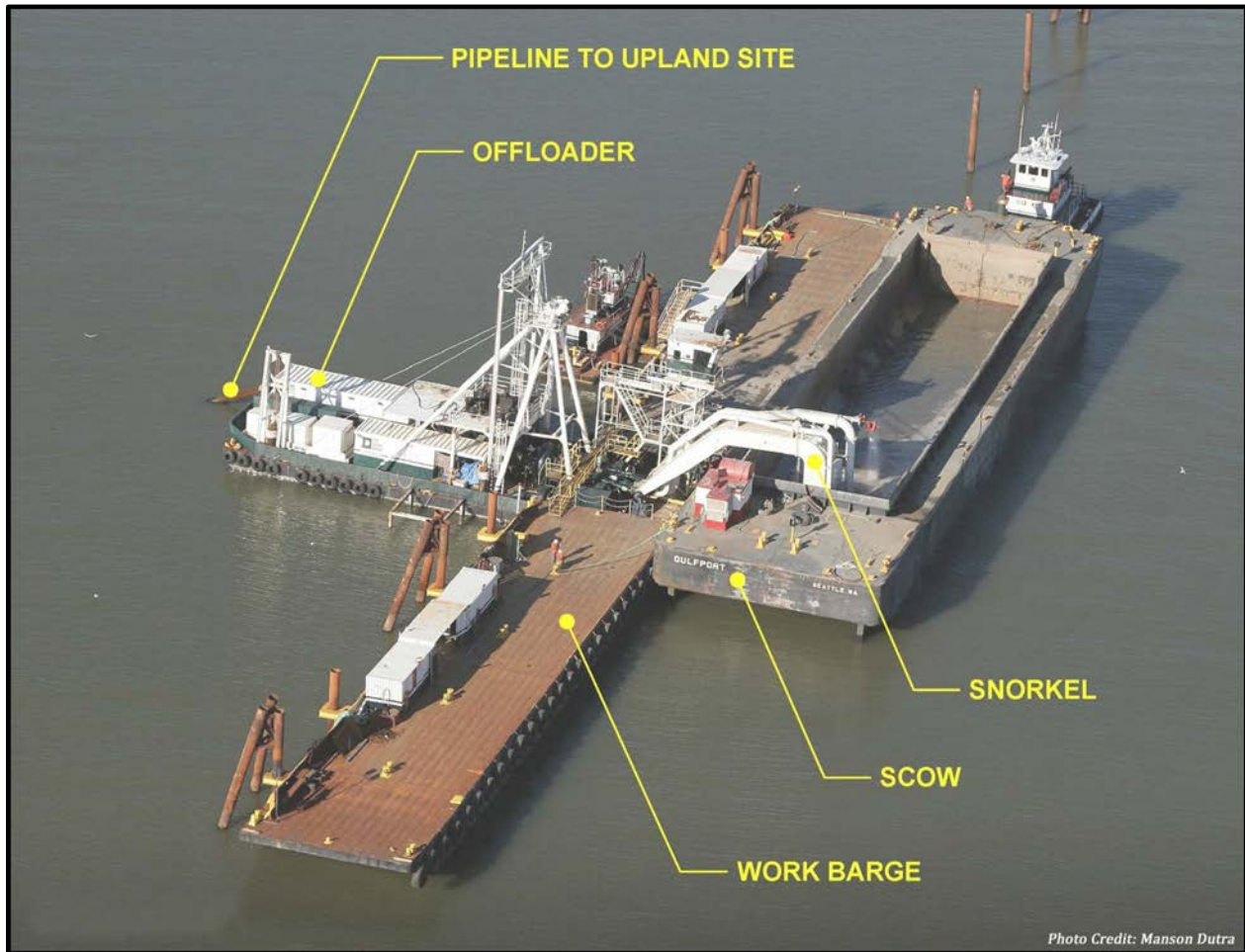
Figure 4-6. Typical Offloader Facilities
