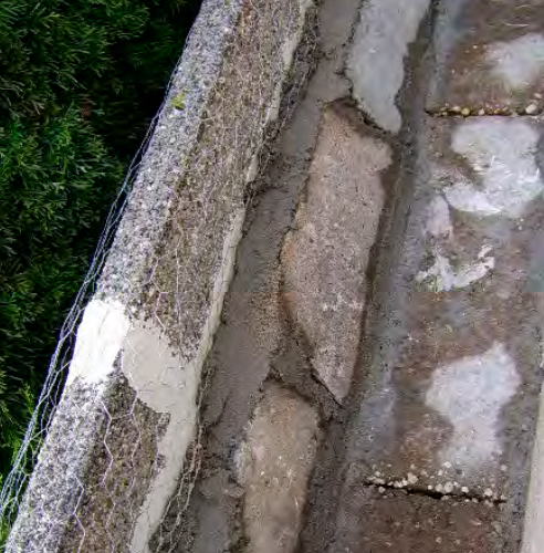
Mortared fillet with chicken mesh
