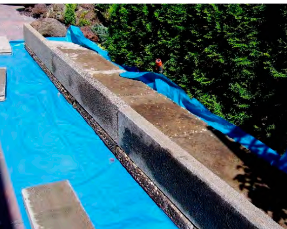
The first course on the gravel tiles
