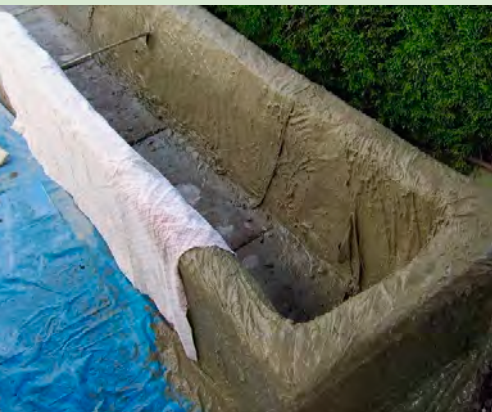
Application of gruel-soaked cloth
