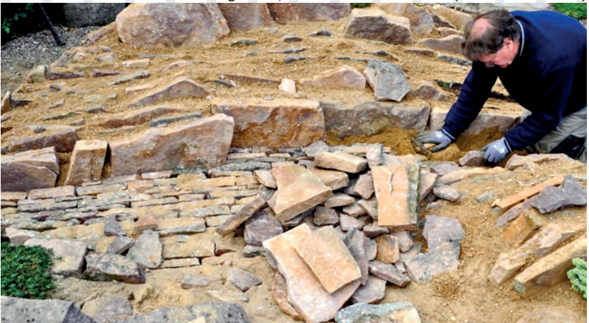
Building rock pavement in Denmark (Kirsten Andersen)
